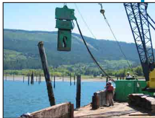
Removal of pilings during Sequim Bay Restoration.
