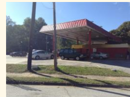
Pure Gas Station-UST
