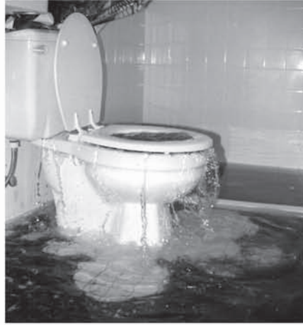
Sewage backing up into a toilet in a house. (Source: U.S. EPA photo)
