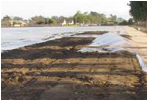
Torn tarps may lead to fumigant gas being released into the air.
