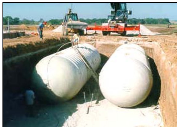
Installation of new USTs - The Seminole Nation (Oklahoma)
