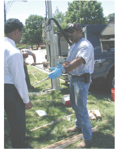
Cleaning up a release at an underground storage tank site
