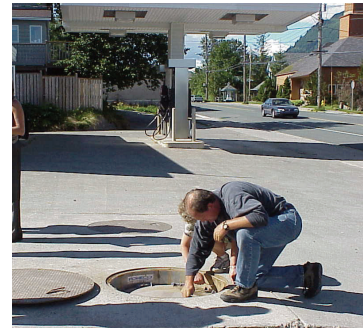
Inspecting a sump
