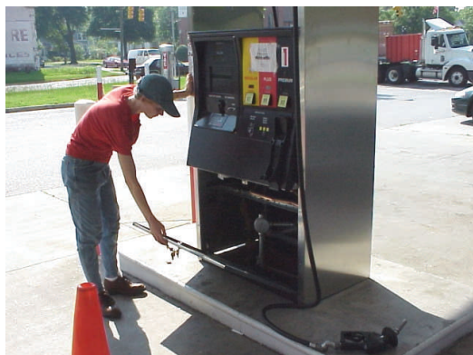
Inspecting beneath a dispenser
