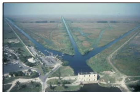
FIGURE 11. An extensive system of canals, levees, and water control structures has modified Everglades water conditions and provides a conduit for pollutant transport. The S-9 pump station (foreground) discharges untreated stormwater from an urban basin into the Everglades (background).
