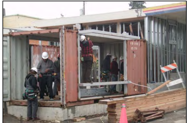
Construction underway using recycled shipping containers (Source: Nye Architecture, LLC)
