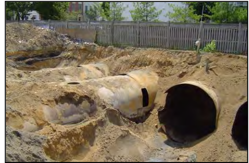
Twenty-eight USTs were excavated and removed from the site during cleanup
