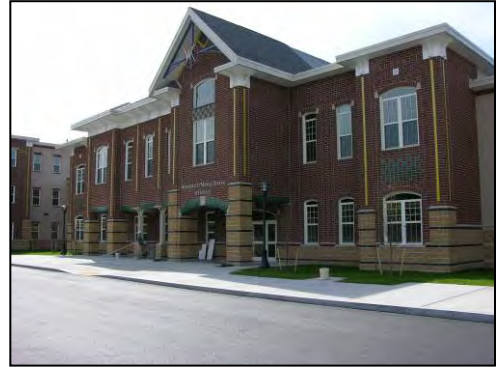
Woonsocket Middle School in Rhode Island
