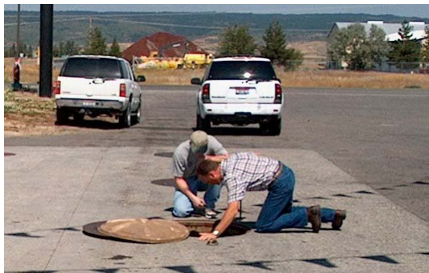
Inspecting a tank sump
