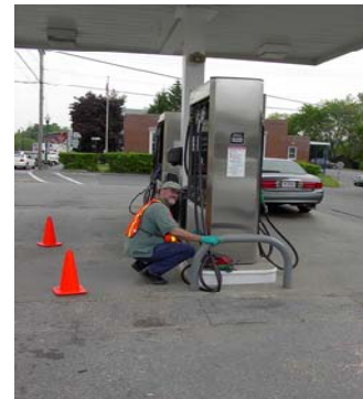
On-site inspection at a tank facility in Maine
