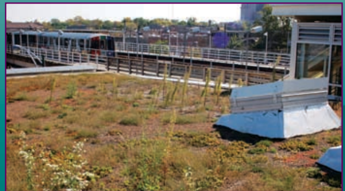
Bethel Center's green roof reduces stormwater runoff, and photovoltaic cells provide clean energy. The center also provides direct access to the Green Line "EI" stop through a connecting bridge.
