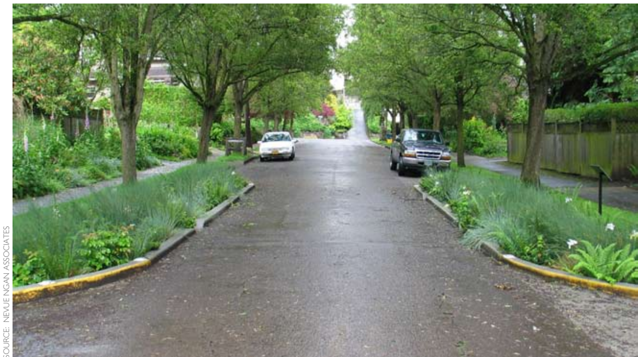
Figure 5-9: A pair of stormwater curb extensions used in a residential street's parking zone in Portland, Oregon.
