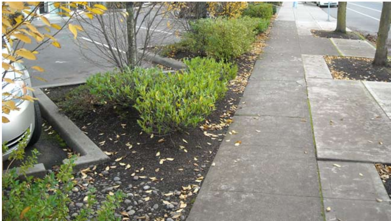
Figure 5-65: This parking lot with angled parking has a series of curb cuts that allow stormwater runoff to enter a landscaped area.
