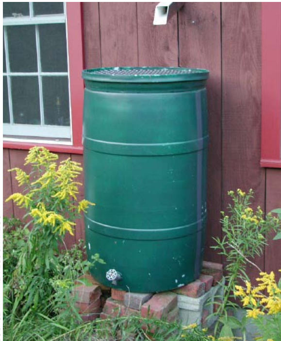
Figure 4-23: Simple residential rain barrels are commonly used to capture and reuse rainwater for irrigation during dry periods.
