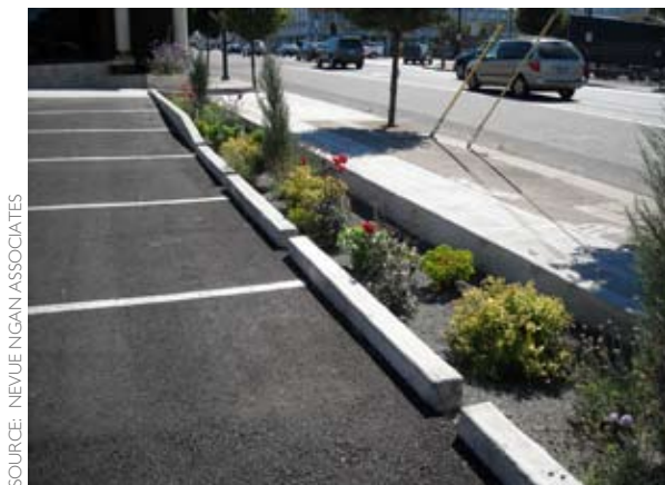
Figure 4-36: A narrow stormwater planter on the edge of a parking lot.
