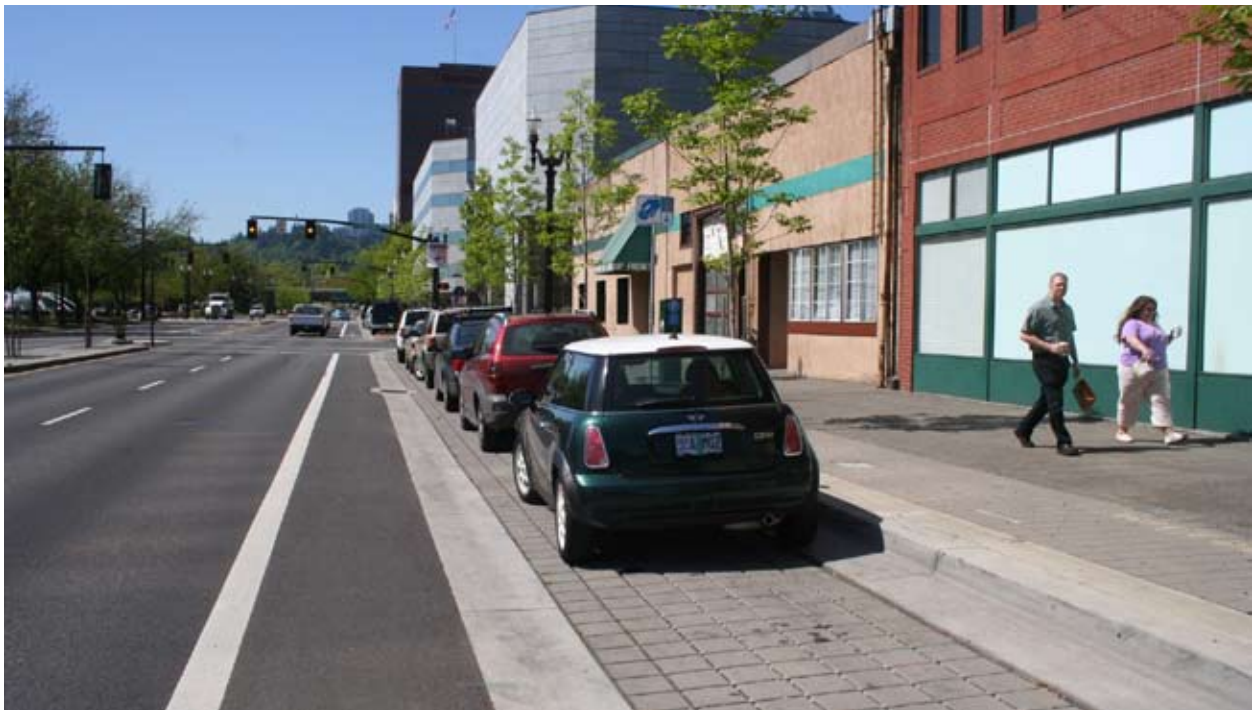
Figure 5-41: This urban street in Portland, Oregon uses pervious paving in its parking zone and could have provided more stormwater management by adding stormwater curb extensions.
