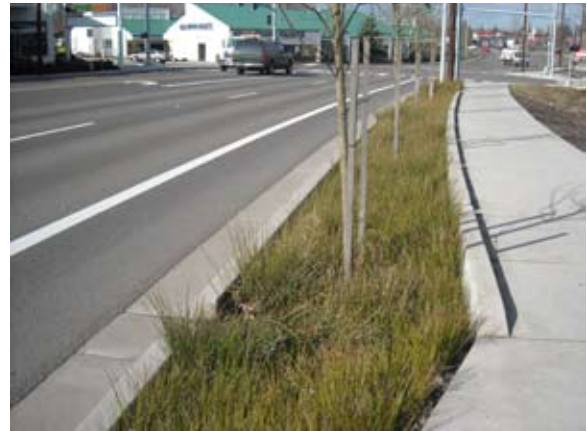
Figure 5-56: Stormwater side swale with bike lanes on arterial street in Oregon City, Oregon.
