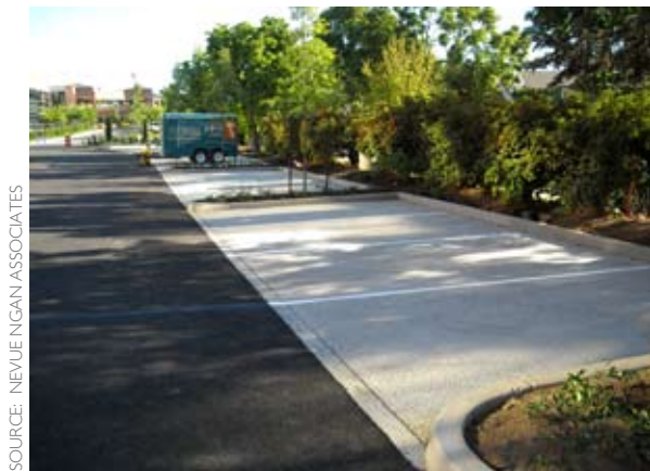
Figure 4-16: Pervious concrete's light color helps reflect heat rather than absorb it.
