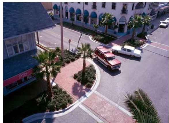
Figure 4-50: Curb extensions can fit nearly anywhere and help calm traffic to protect pedestrians.
