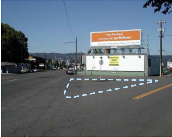
Figure 4-41: Large under-used areas of asphalt can easily be converted into infiltration gardens.
