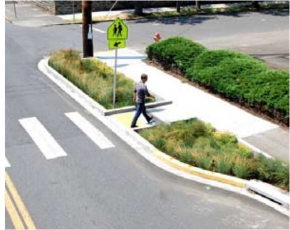
Figure 4-54: Accessible pedestrian ramps can also be integrated into the design of stormwater curb extensions.
