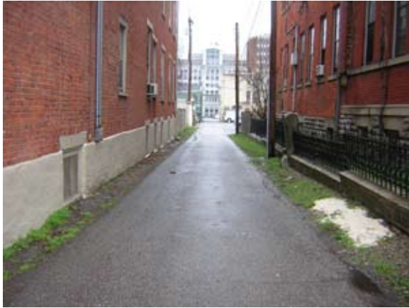
Figure 5-48: EXISTING: An existing urban alley in downtown Covington.
