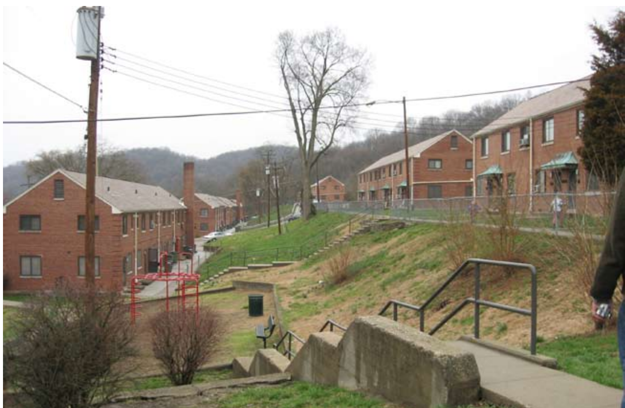
Figure 6-10: The existing conditions at the Latonia Terrace site in Covington, Kentucky.
