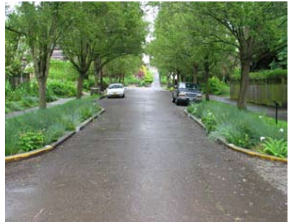
Figure 4-55: A pair of stormwater curb extensions installed along a neighborhood street.
