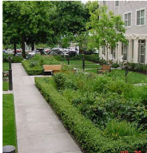
Figure 4-44: An infiltration garden installed within an apartment complex in Portland, Oregon.
