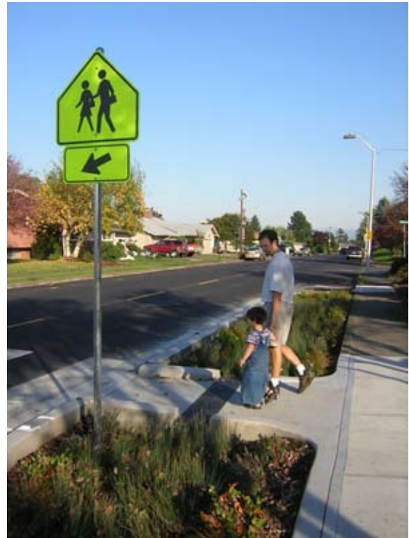
Figure 4-49: Curb extensions can provide stormwater management opportunities and safer crossings for pedestrians.
