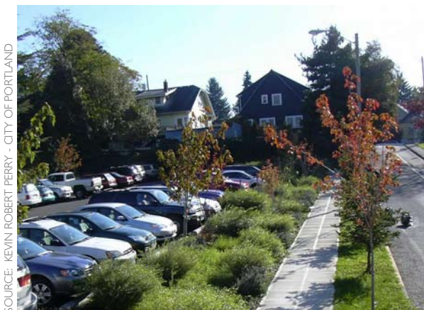
Figure 4-29: An elementary school parking lot with a stormwater swale.
