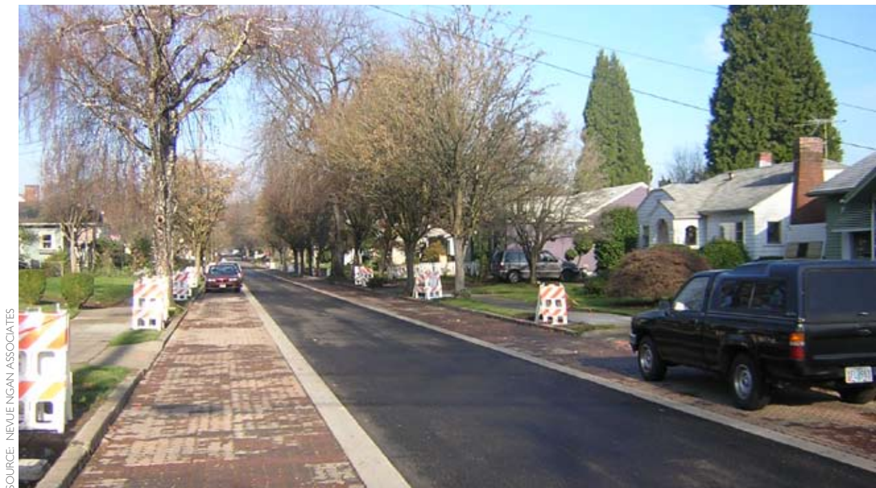
Figure 5-21: Pervious paving used in a residential street's parking zone. Notice the visual "narrowing" of the street.
