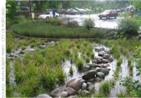
Figure 5-70: This infiltration garden captures, slows, absorbs, and filters runoff from a nearby street and parking lot.
