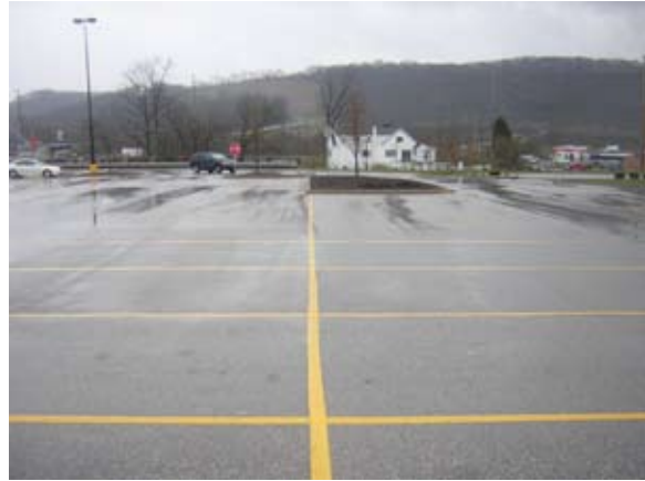
Figure 4-30: These parking spaces could be made just a few feet shorter to provide room for swales between rows of parked cars.
