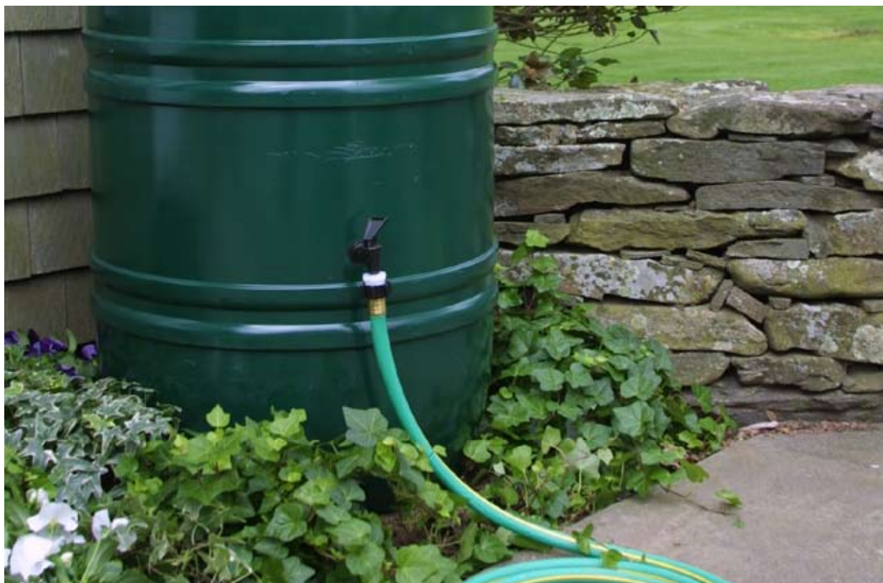
Figure 4-21: Residential rain barrels used for summertime irrigation.
