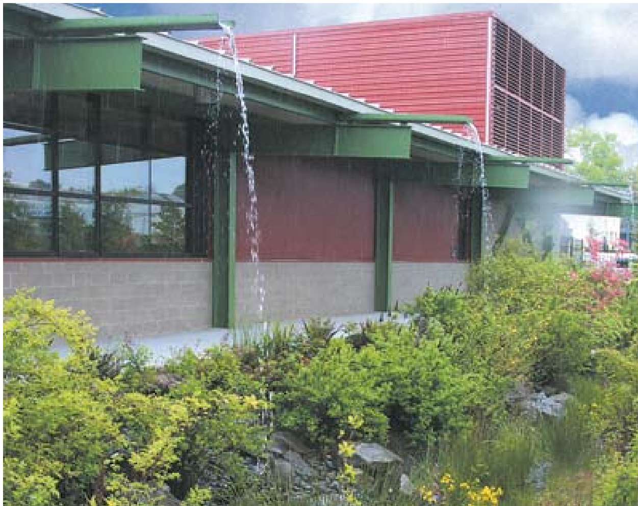
Figure 4-60: An example of allowing water to cascade from a building rooftop into a landscaped area.
