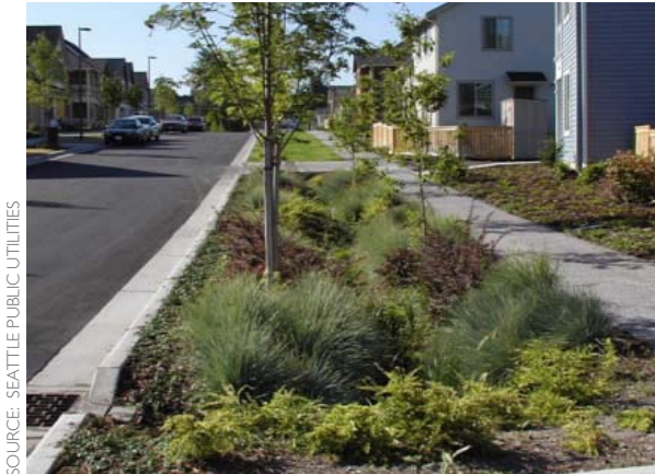
Figure 4-27: A residential street with a stormwater swale.
