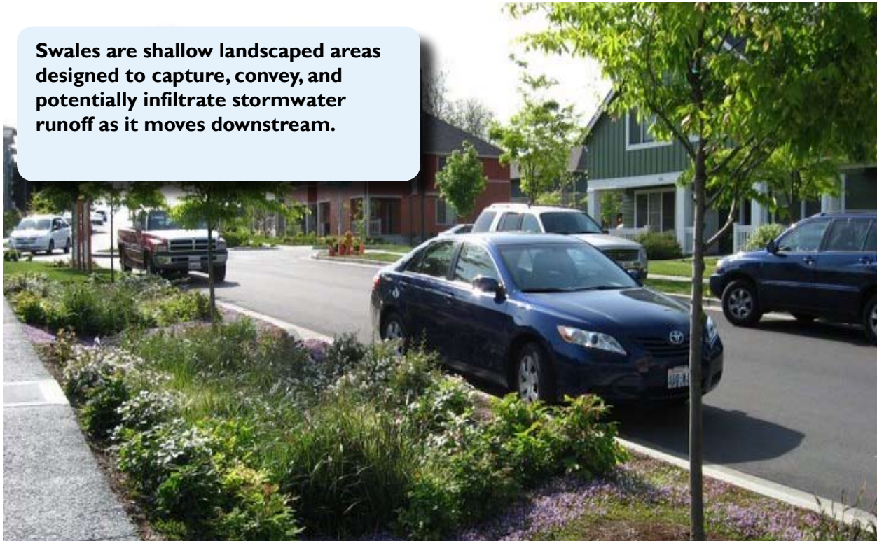
Figure 4-25: A new residential street incorporates a stormwater swale to collect stormwater runoff in Seattle, Washington.
