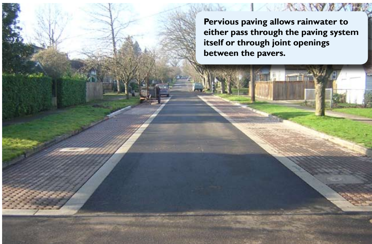
Figure 4-6: Pervious paving used in the parking zone on a residential street in Portland, Oregon.
