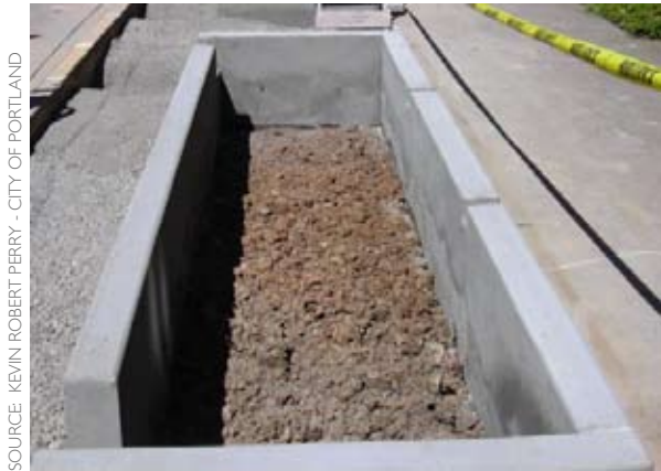
Figure L-1: Native soil is rototilled to break up construction compaction.
