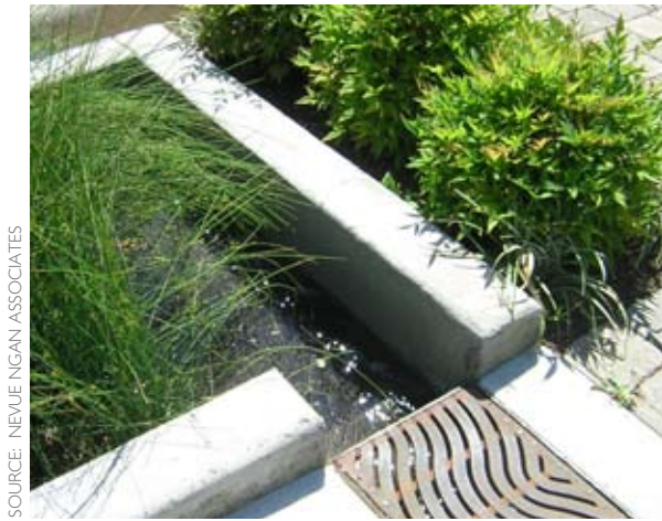
Figure J-2: A small, 18"-wide sediment forebay at the entry curb cut of a street stormwater planter.
