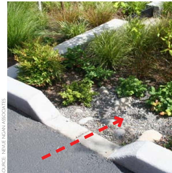
Figure H-3: A standard curb cut allows stormwater runoff to enter a parking lot rain garden. This curb cut has 45 degree chamfered sides.
