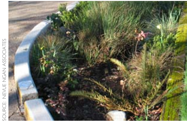
Figure J-1: A sediment forebay in a stormwater curb extension.
