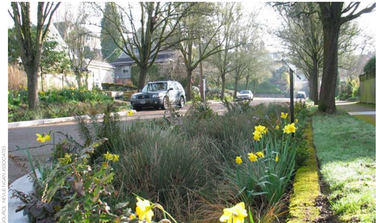
Figure F-2: This stormwater curb extension was built to save both the existing curb of the street as well as the 30-year old ornamental pear trees.
