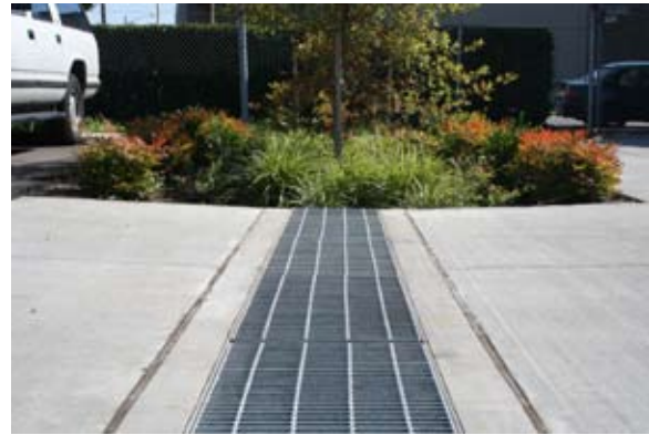
Figure I-1: This trench drain example connects two stormwater facilities in an industrial parking lot site.
