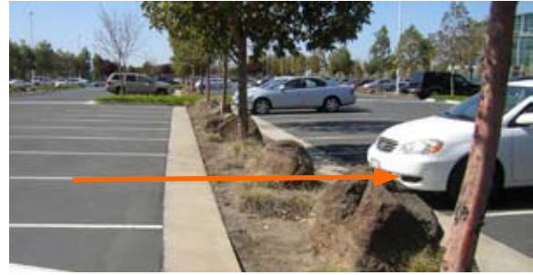
Figure D-5: Failed pedestrian circulation in a parking lot. Due to poor design, people have trampled this vegetated swale to the point where the landscape cannot grow.
