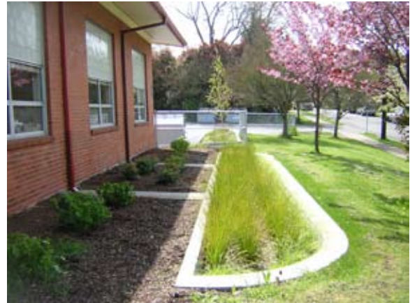
Figure M-1: In this scenario, the infiltration planter is offset 8' from the building edge.
