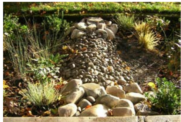
Figure E-5: Simple check dams made of stacked rocks or gravel can be used on mildly sloped stormwater facilities.
