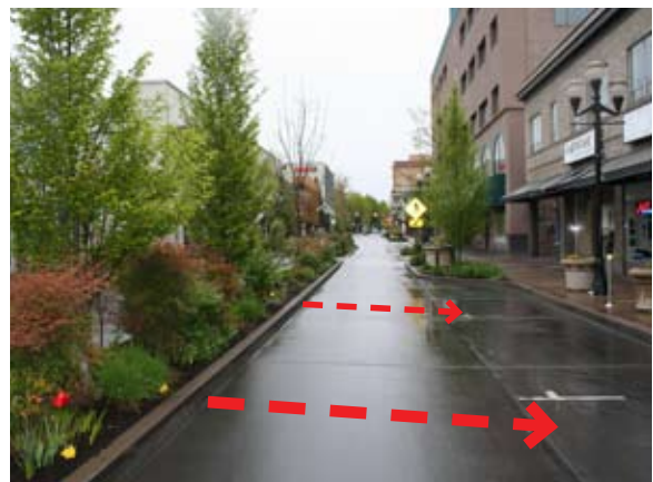
Figure C-7: This crowned street has a landscaped center median. Unfortunately, stormwater runoff is directed away from it.
