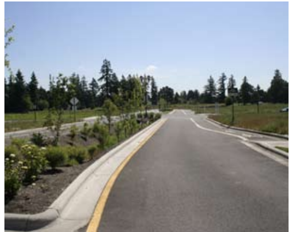
Figure C-5: This new green street is designed as a reverse crowned street, allowing runoff to flow into a center median vegetated swale.
