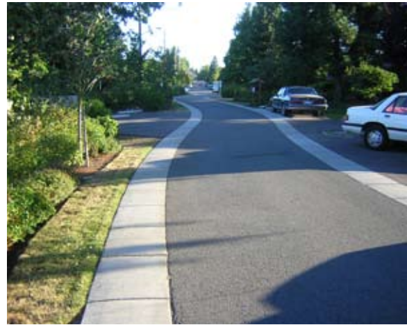
Figure G-1: This “curbless” street example allows sheet flow of runoff into a vegetated swale.
