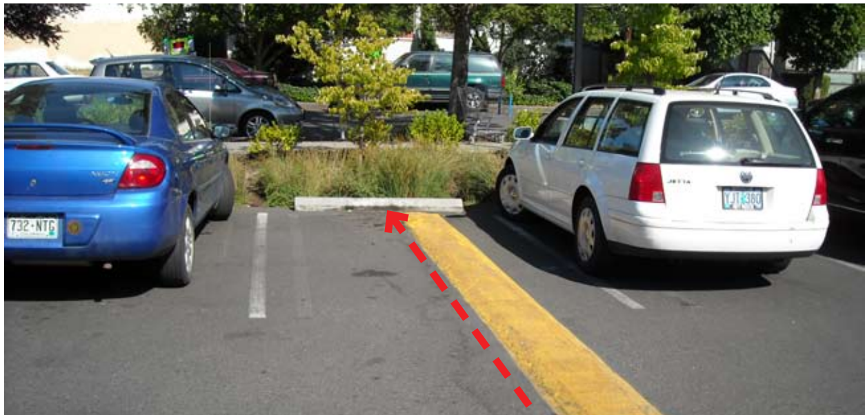
Figure I-3: This asphalt speed bump redirects stormwater into a vegetated swale. Without the speed bump, stormwater runoff would enter the vegetated swale much lower in the system, bypassing some of the area available for treatment.
