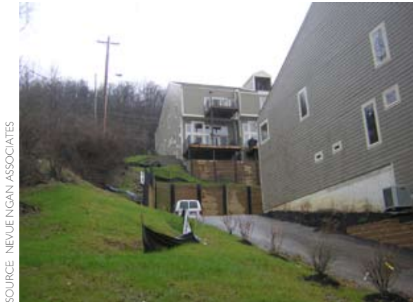
Figure E-1: A steep site condition in Northern Kentucky.
