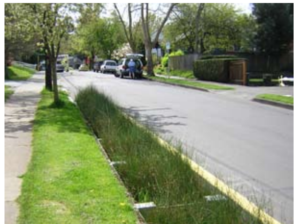
Figure C-6: This green street retrofit is designed with a narrow curb extension that captures runoff from an existing crowned street.
