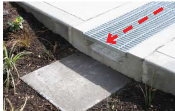
Figure I-2: A concrete unit paver is placed at the exit point of this trench drain. The pad helps dissipate water velocity as it drops from the trench drain to the finish grade of the stormwater facility.
