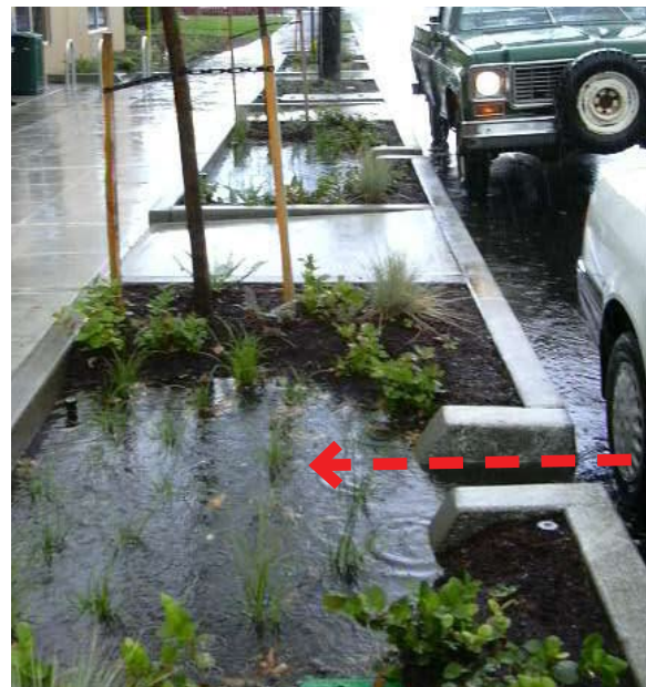
Figure H-6: A standard curb with wings allows stormwater runoff to enter a stormwater facility. The wings help retain the side slope grade on each side of the curb cut opening.
