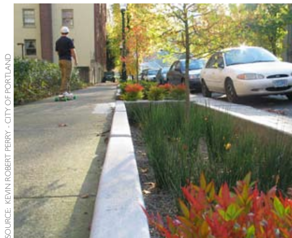
Figure L-3: A 2" layer of pea gravel mulch is applied to a stormwater planter.
