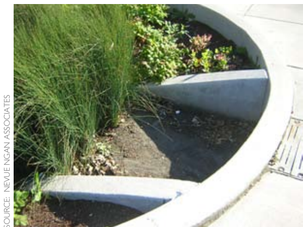
Figure J-3: A 3x3' concrete pad is used as a sediment forebay for a large street rain garden. The plant material acts as a dam, allowing debris to settle on the pad for regular removal.
