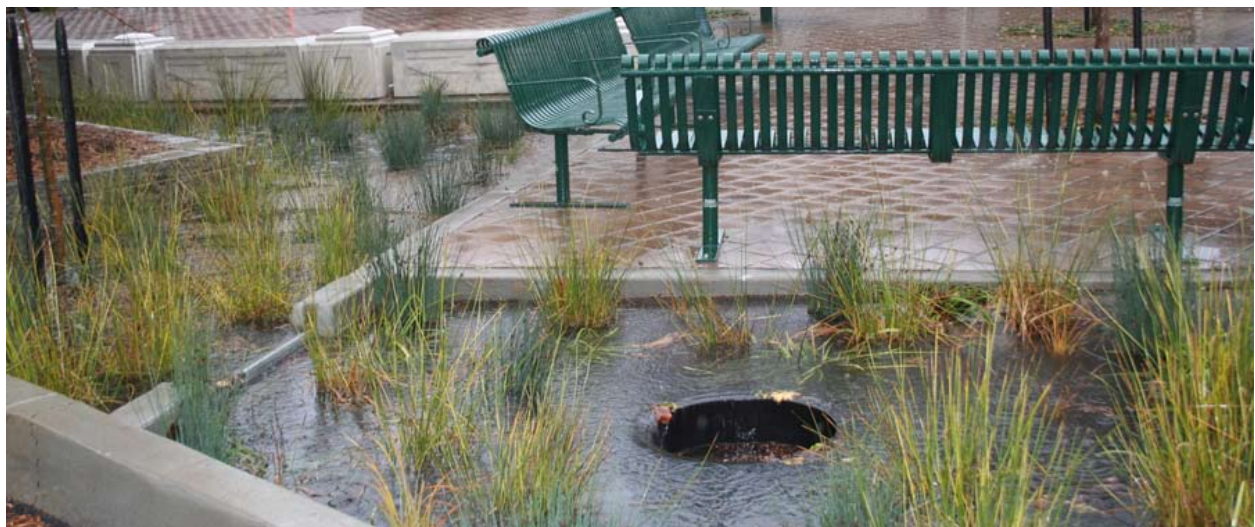
Figure K-3: An adjustable weir retains stormwater to an 8" depth within this vegetated swale before overflowing into the storm system.
