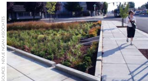
Figure D-3: A perimeter concrete curb was installed around this urban rain garden to help protect both pedestrians and the stormwater facility.
