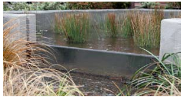
Figure E-4: This adjustable weir can control how much water is to be retained in a rain garden.
