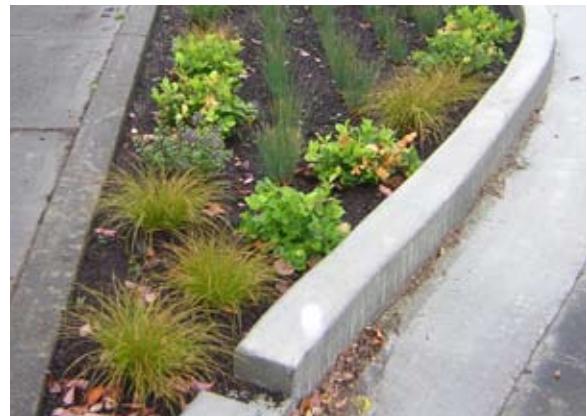
Figure K-2: Overflow from a mid-block stormwater curb extension exits from a curb notch and flows back onto the street.
