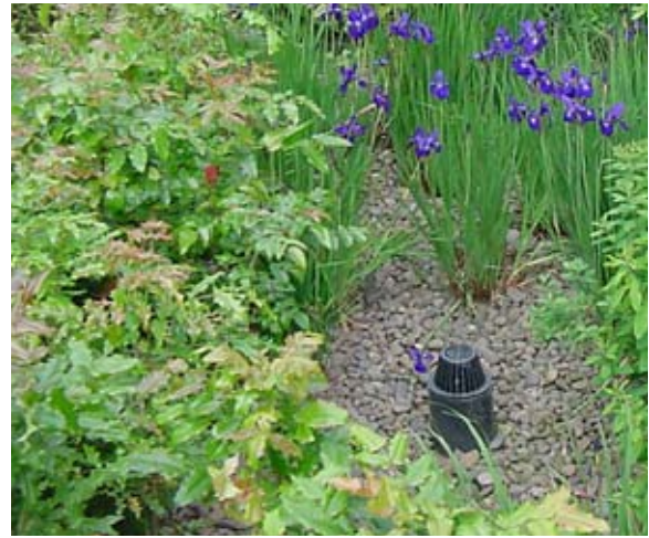
Figure K-1: Overflow from this rain garden enters a 4" riser connected to the storm system.
