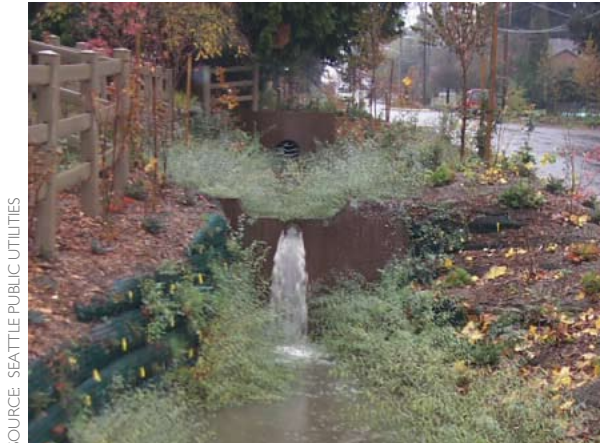
Figure E-2: Terraced concrete weirs allow a vegetated swale to be graded with a much shallower slope than the adjacent street's grade.
