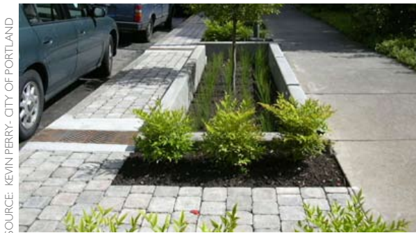
Figure D-1: This street that uses stormwater planters adjacent to on-street parking and provides a 3-foot walkway that allows people to access the sidewalk and parking zone.
