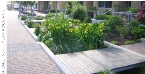
Figure D-2: A series of “stormwater bridges” allows people to cross over a vegetated swale.
