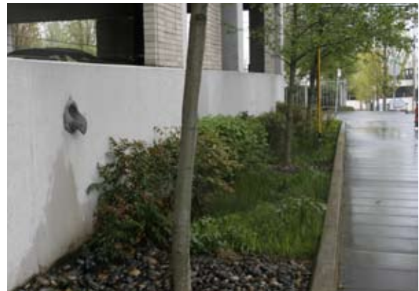
Figure M-2: A plastic liner is adhered to the building foundation, but runoff can still infiltrate.
