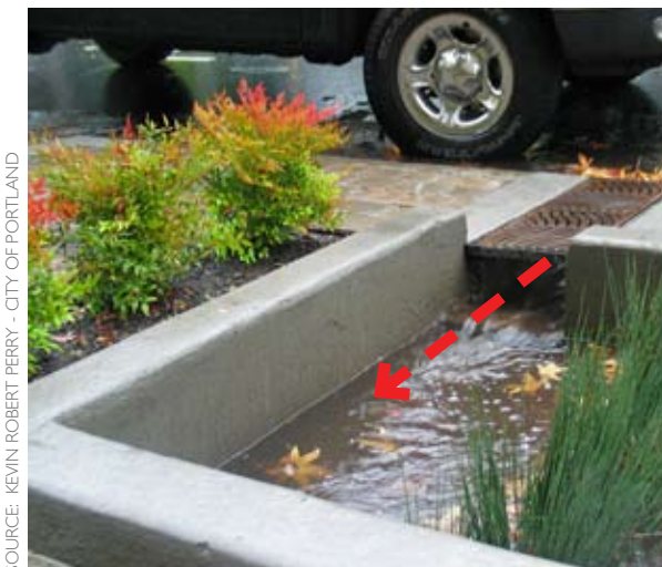
Figure H-9: A grated curb cut allows stormwater to pass under a street stormwater planter's pedestrian egress zone.
