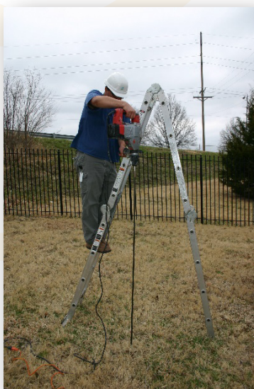
Figure 1: Vapor Probe Installation
