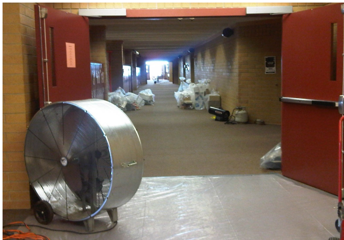
Venting of hallway.
