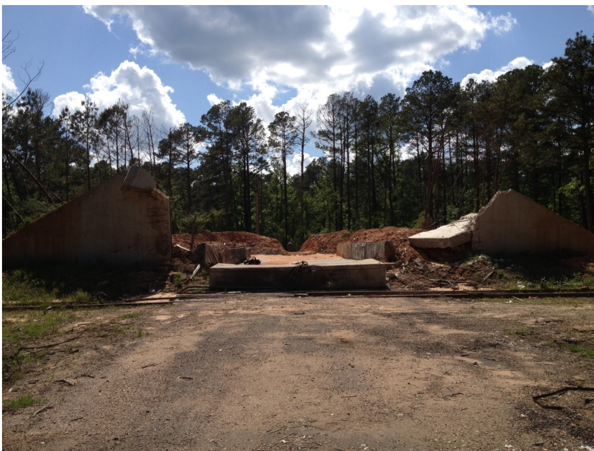
Photo 3: Result of explosion of magazine storing black powder and tractor trailers storing M6 Propellant in October 2012
