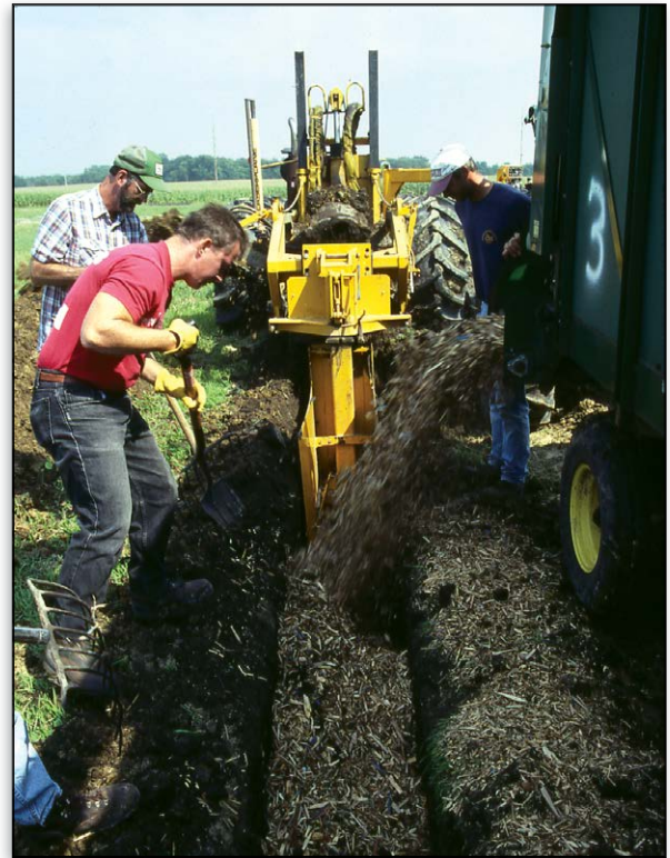
Denitrifying bioreactors, like this one in Iowa, may operate for a decade without maintenance.
