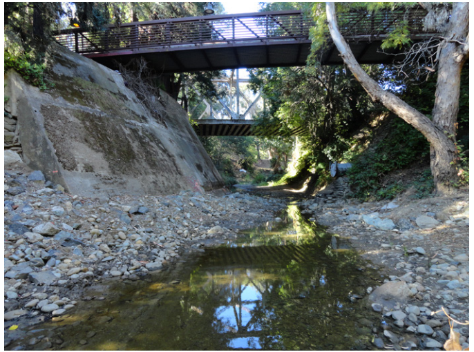
San Francisquito Creek after Bonde Weir removal, 2013. Photo: Joe Issel.
