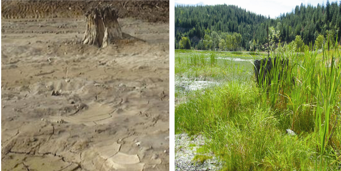
Figure I-2: Before and after photographs of the Bunker Hill Superfund Site in Idaho where contamination was left on-site and capped with biosolids compost and wood ash. A long-term O&M plan was established to ensure that attractive nuisance (see definition on page 3-2) issues did not result. See Appendix A for additional information. Photographs courtesy of Dr. Sally Brown, University of Washington.
