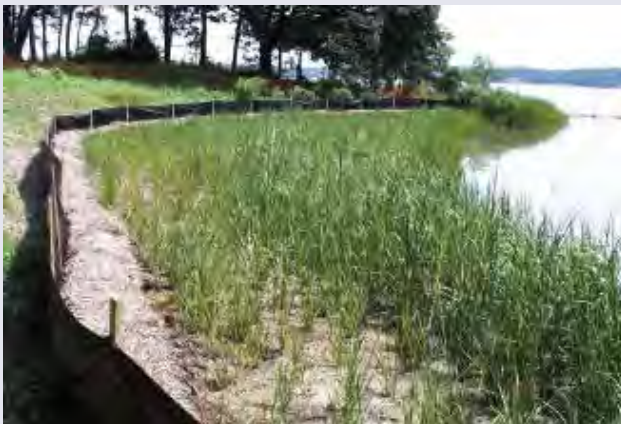
Figure 13. Newly planted marsh with fiber logs allowing plants to establish root system and stabilize shoreline. Source: VIMS, 2006.
