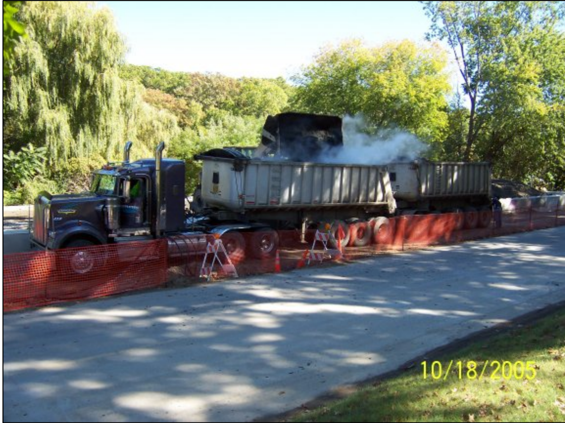
Figure 3-5 Loading treated sediment for transportation to the Ottawa Farms landfill
