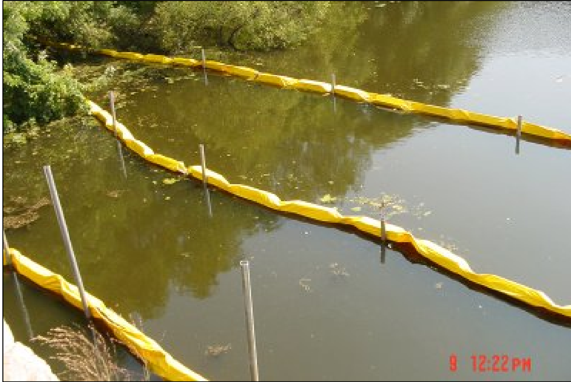
Figure 2-10 Isolation of Ruddiman Pond work areas using multiple silt curtains
