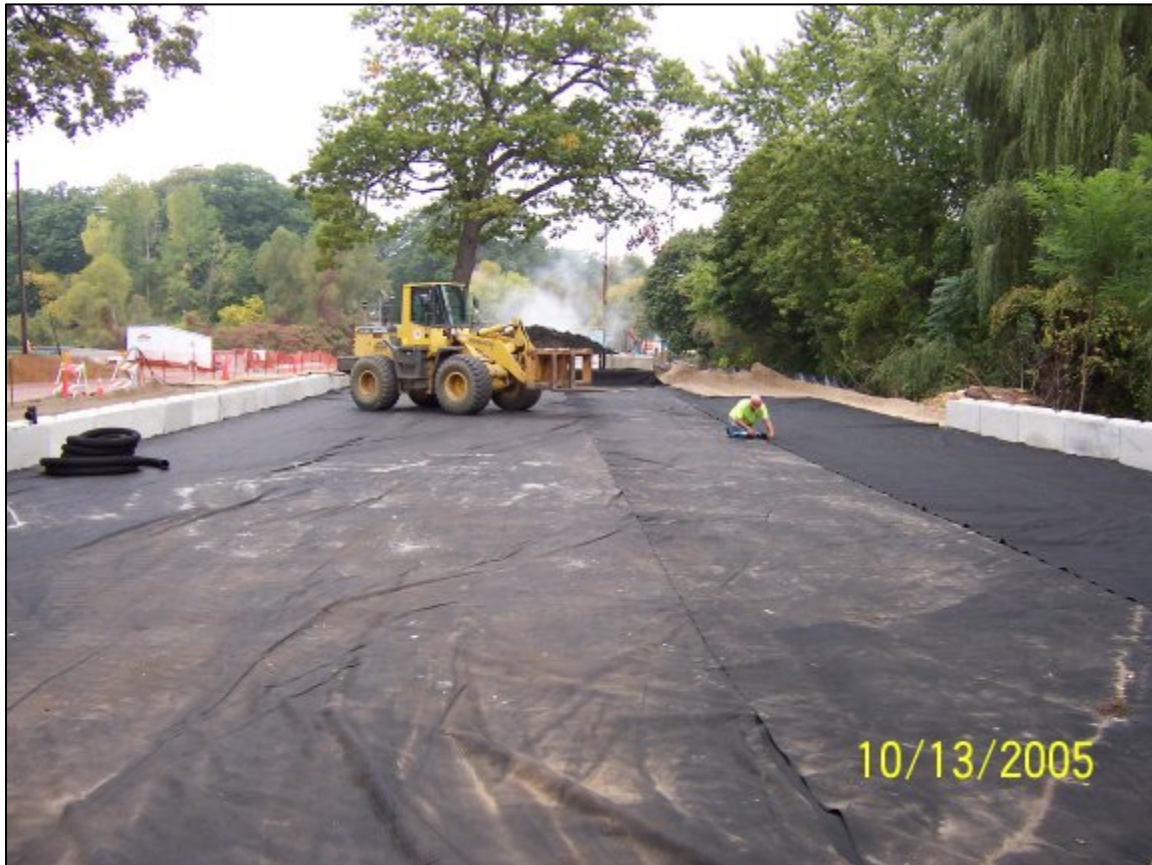
Figure 2-9 Sediment dewatering pads
