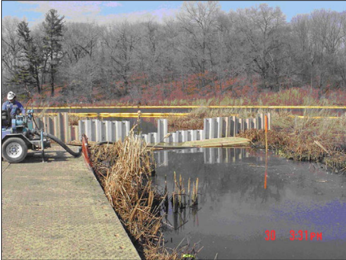
Figure 2-6 Sheet piling isolating a portion of a creek channel
