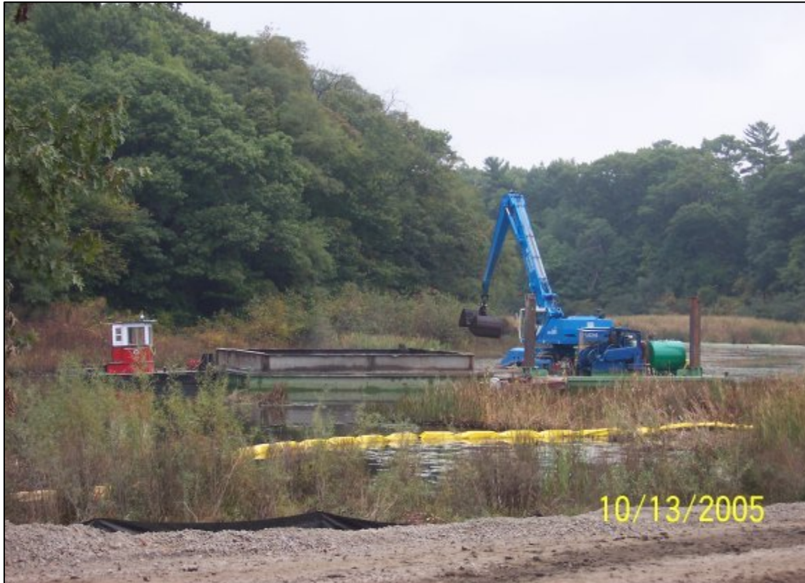
Figure 3-1 Tug and barge dredging operations within the Ruddiman Pond remediation area
