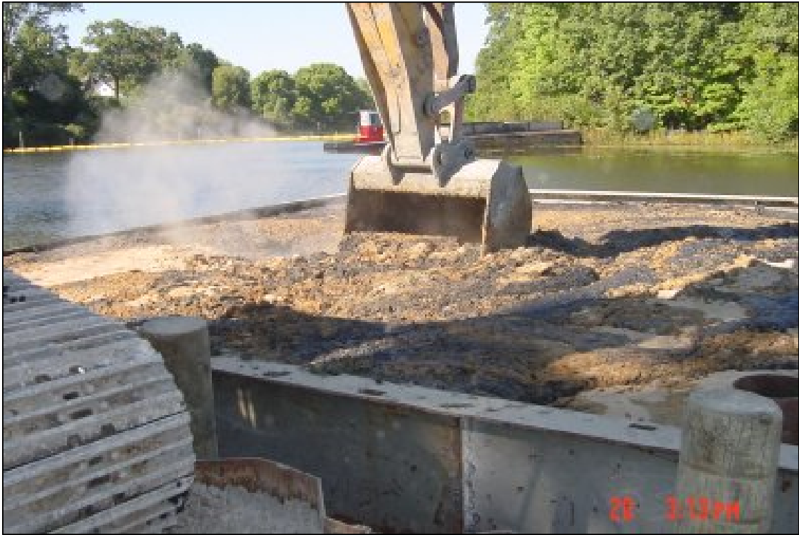
Figure 3-4 Addition of Calciment ® to sediments on the dredging barge
