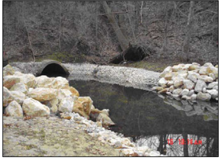
Figure 2-5 Headwater dissipation structure
