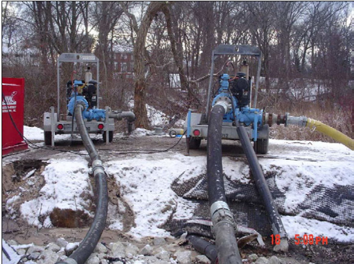
Figure 2-8 By-pass pumping around Areas D and C
