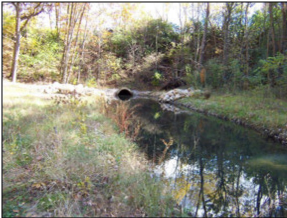
Figure 9-1 Appearance of Ruddiman Creek Main Branch remediation area six months after completion of remediation project
