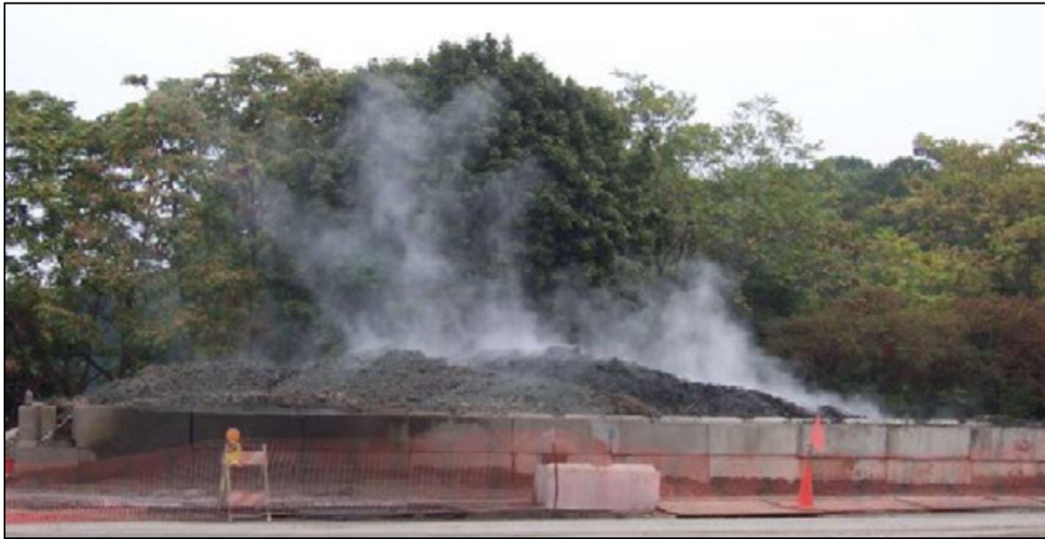
Figure 3-3 Sediments mixed with Calciment® in the drying bed
