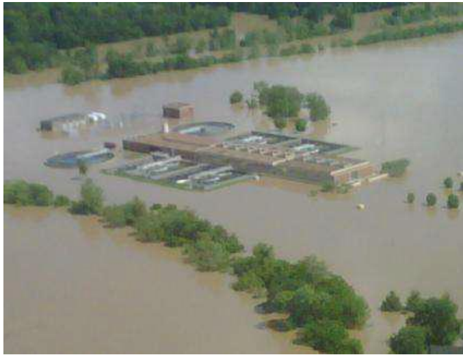
Flooding at Nashville's Metro Water Service's K. R. Harrington Water Treatment Plant on May 2, 2010 knocked the plant out of service. (Source: Metro Water Services)
