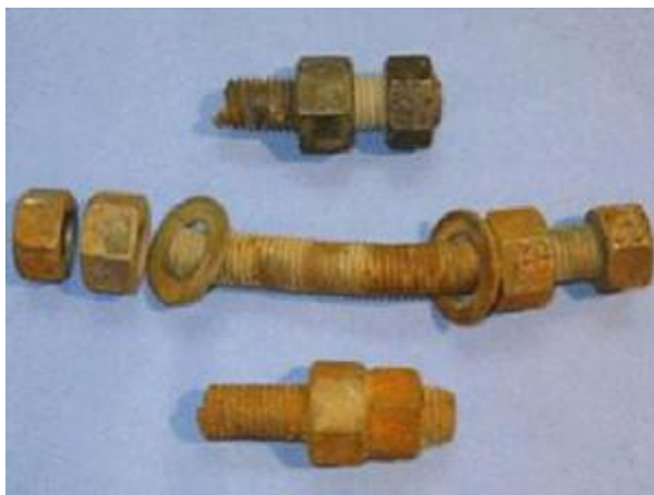
A failure of bolts at a pipe joint is believed to have caused the water MWRA water main break. (Source: MWRA)
