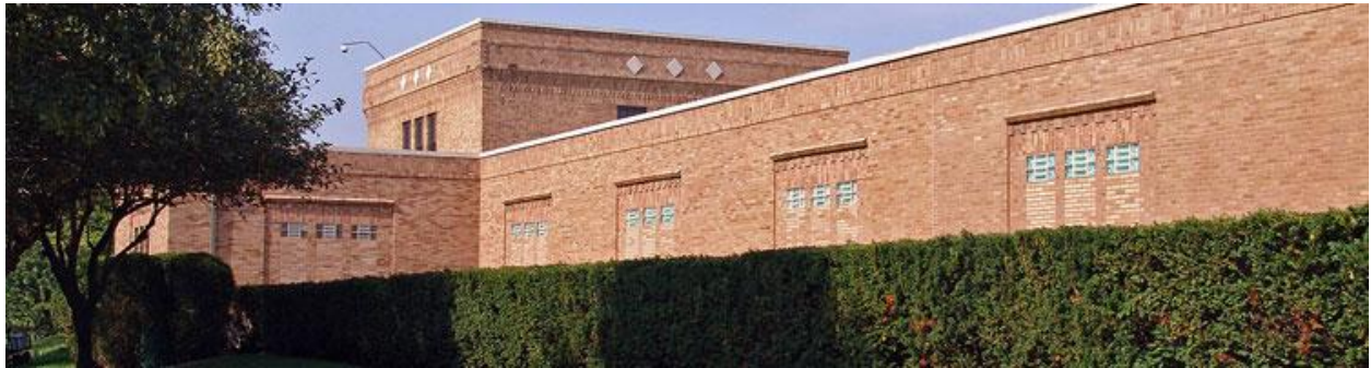
City of Evanston, Illinois water treatment plant.
