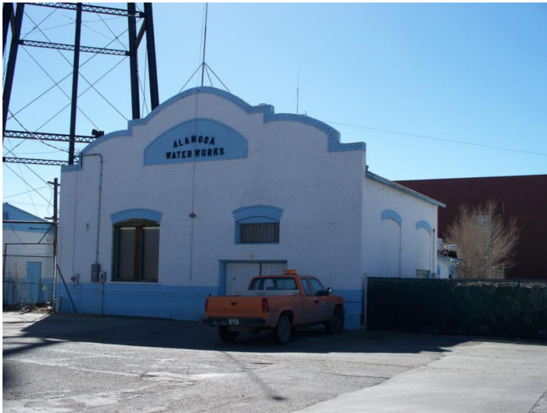
The water works for the city of Alamosa, Colorado. (Source: Colorado Department of Public Health and Environment)
