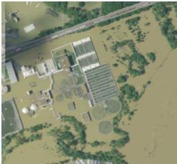
Flooding from the Cumberland River overwhelmed Nashville's Metro Water Service's Dry Creek Wastewater Treatment Plant. (Source: Metro Water Services)
