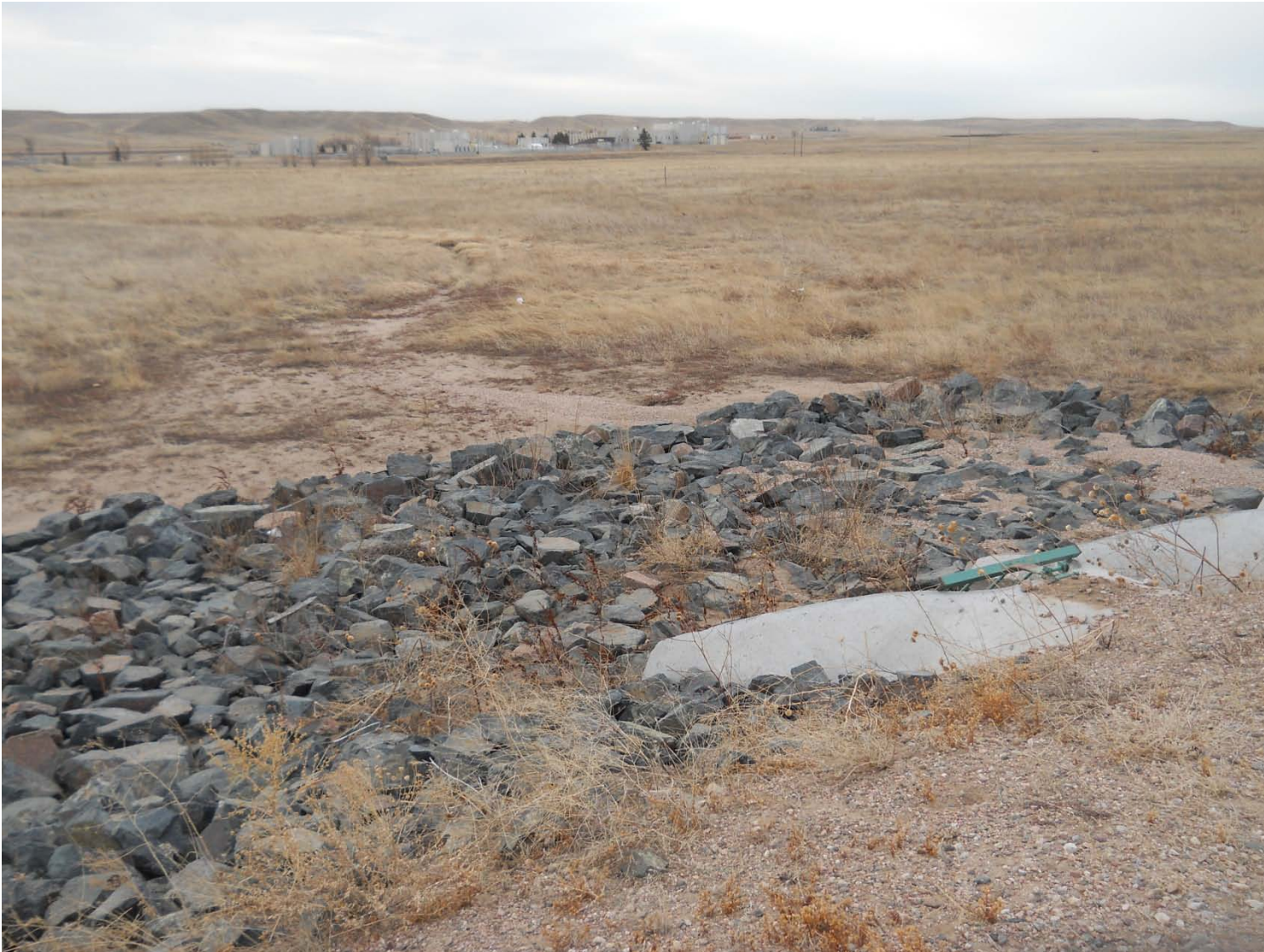
Eastern ditch crossing on access road.
