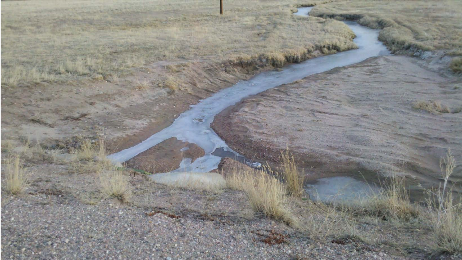
Western ditch crossing on access road.
