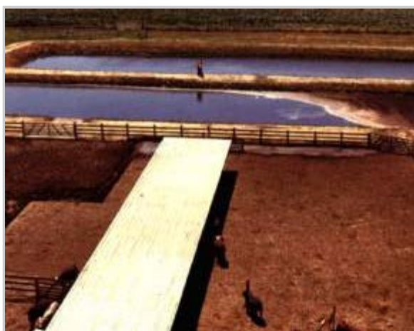
Shed and outside lot with runoff control
