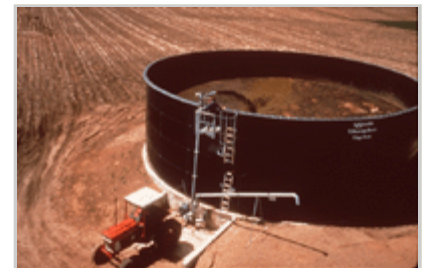
Fabricated steel manure storage
