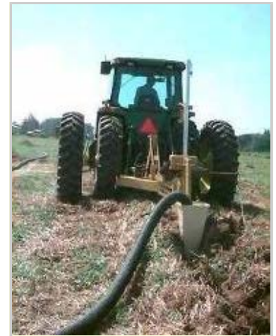
Drainage plow being pulled by farm tractor installing a tileline
