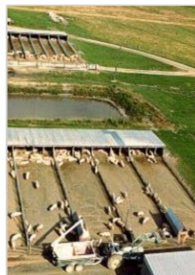
Options for handling manure from open lot holding pond for runoff from outside lot Source: Davis-Purdue Farms
