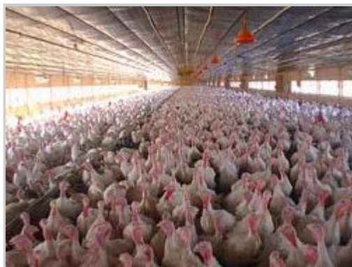
Modern enclosed poultry building Source: Purdue University
