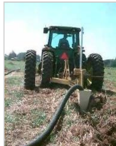
Drainage plow being pulled by farm tractor installing a tileline
