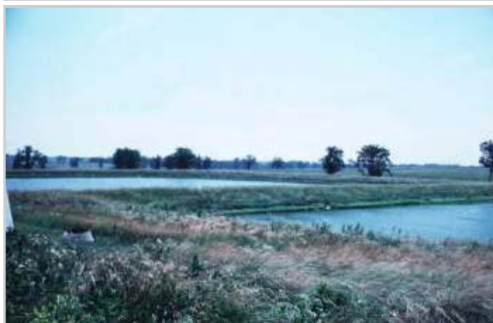
Manure treated and stored in a multi-cell lagoon before land application
