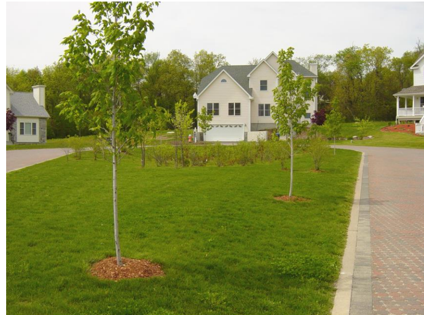
Engineered swales, bioretention basins and porous pavers
