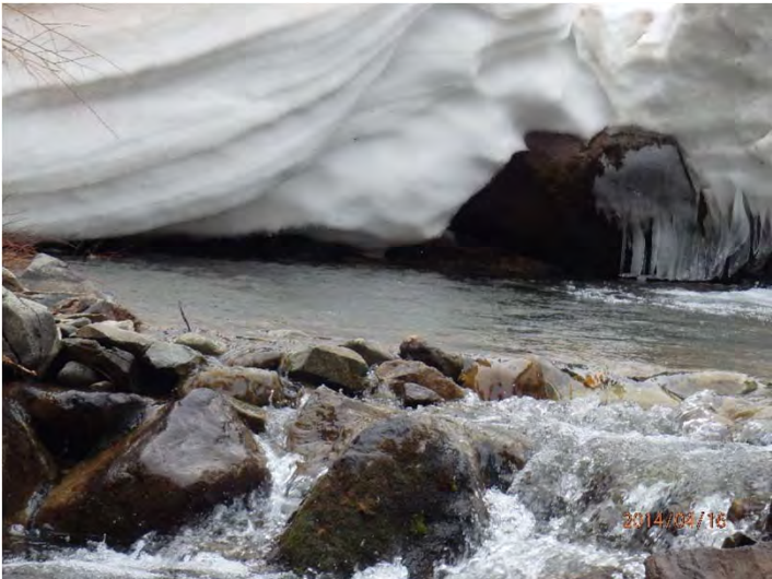
A58 Upstream Culvert
