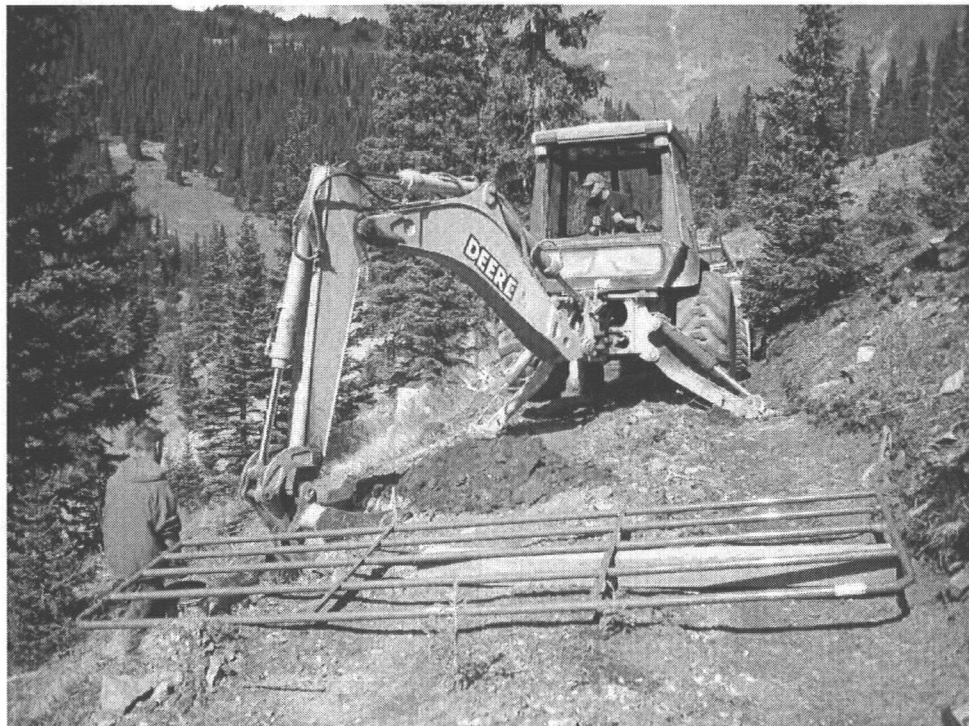
Photo 40 Installation of gate posts on north access road 10/21/10.
