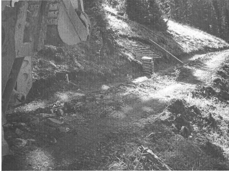
Photo 39 Gate installation materials.
