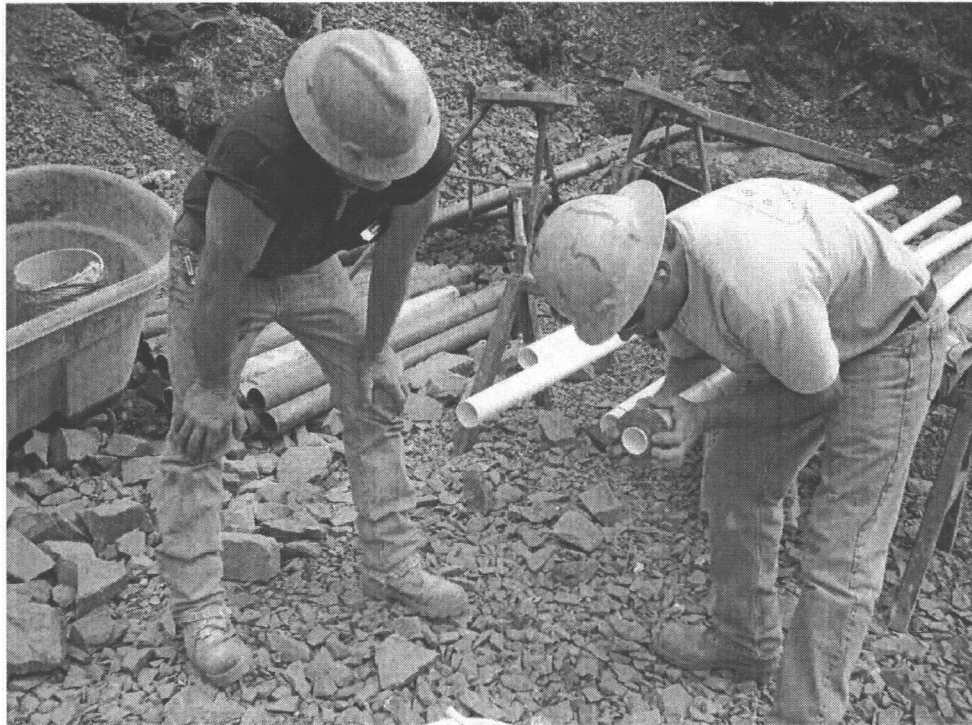
Photo 27 K-packer placement on riser.
