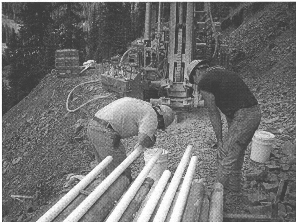
Photo 26 Placement of K-packer on 2" riser.
