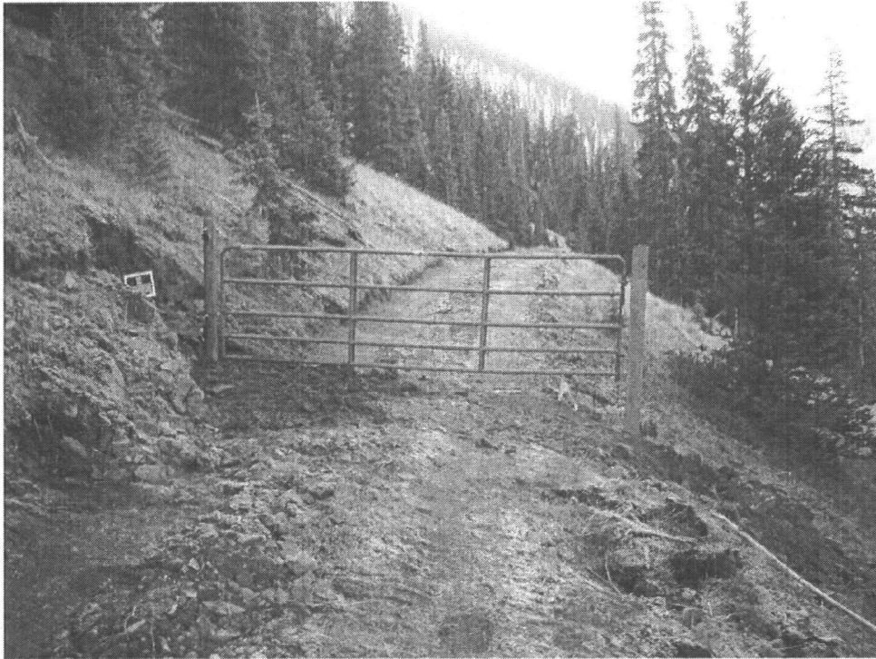
Photo 47 Final gate installation on 10/21/10.
