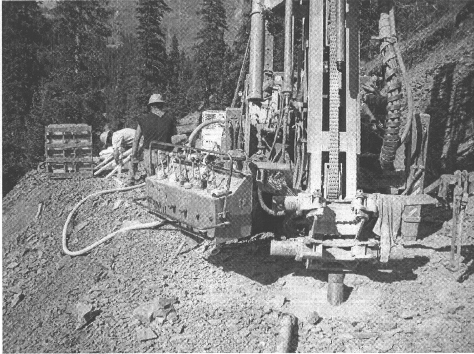
Photo 25 Drilling rig setting up for well construction at RBMW01.
