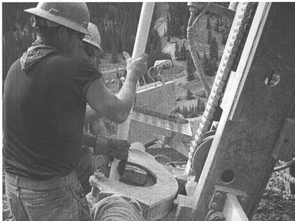
Photo 28 Emplacement of well screen into RBMW01.
