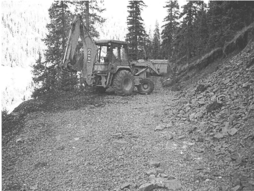
Photo 16 Site cleanup and follow-up excavation work prior to drilling on 09/27/10.
