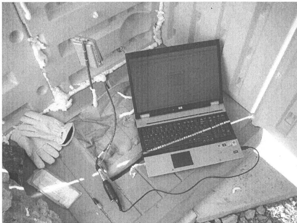
Photo 45 Programming of the pressure transducer at Upper Gold King #7. Note the transducer cabling, and the docking station.
