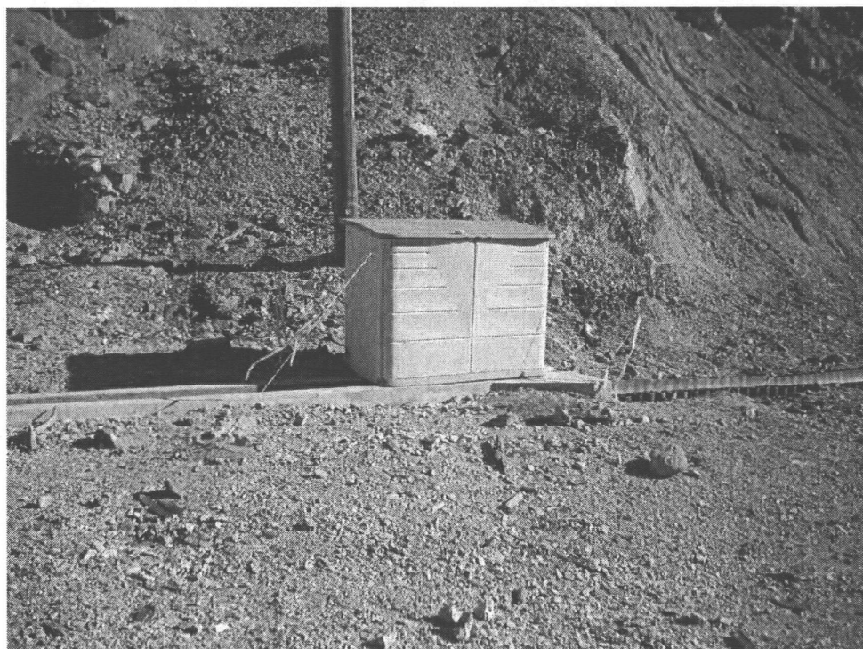
Photo 46 Completed snow shelter at Upper Gold King #7.
