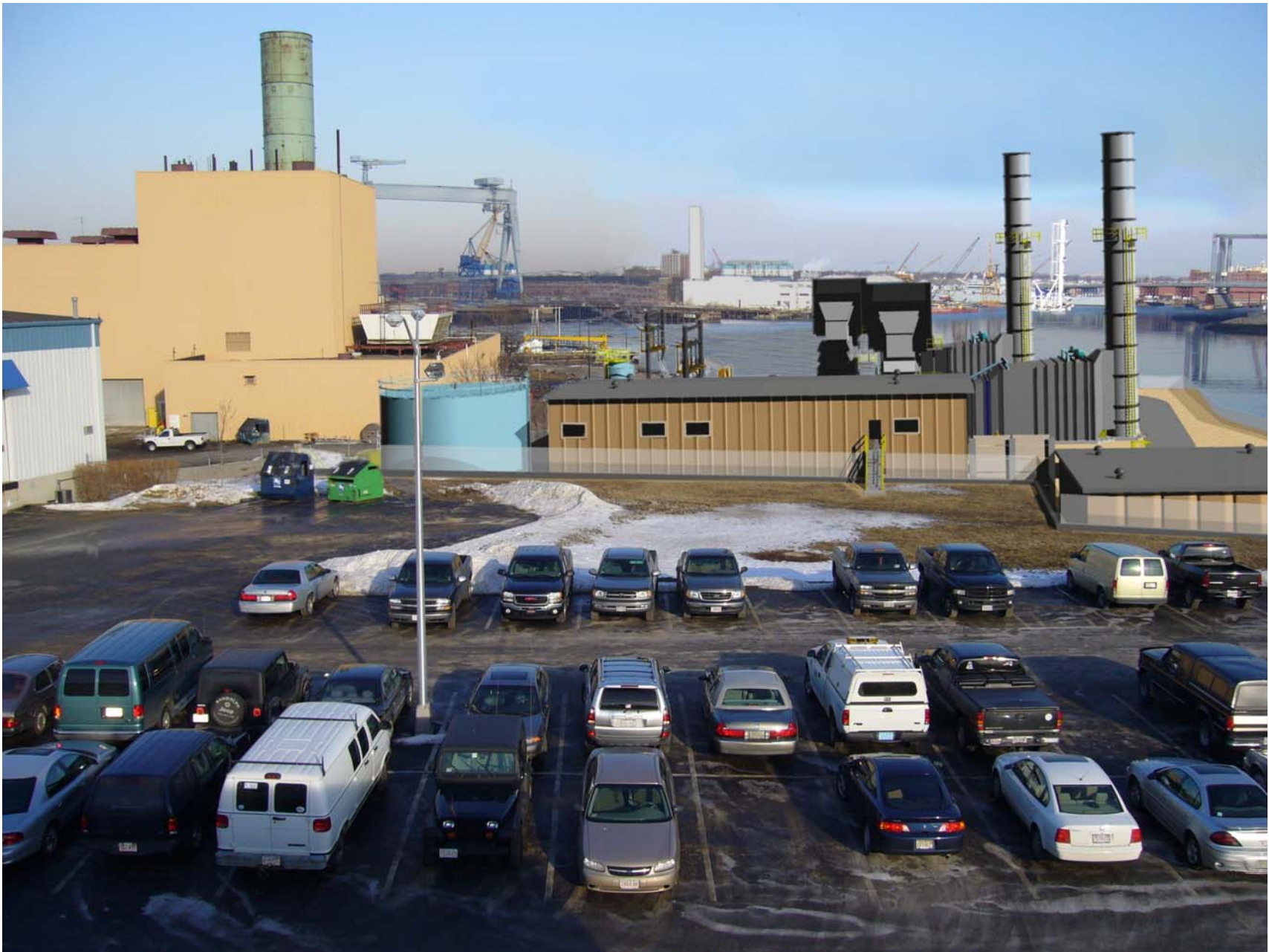
Figure 2-3 Rolls Royce Trent 60 WLE Rendering – View from BELD Offices/Parking Lot Thomas A. Watson Generating Station Braintree, Massachusetts
