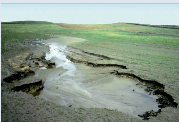
Water runoff eroding a field. (Photo courtesy of USDA/MO NRCS)
