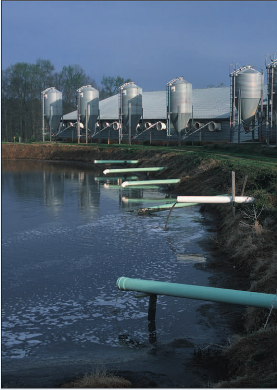
An automated lagoon waste management system for a 900-head hog farm. (Photo courtesy of USDA/NRCS)
