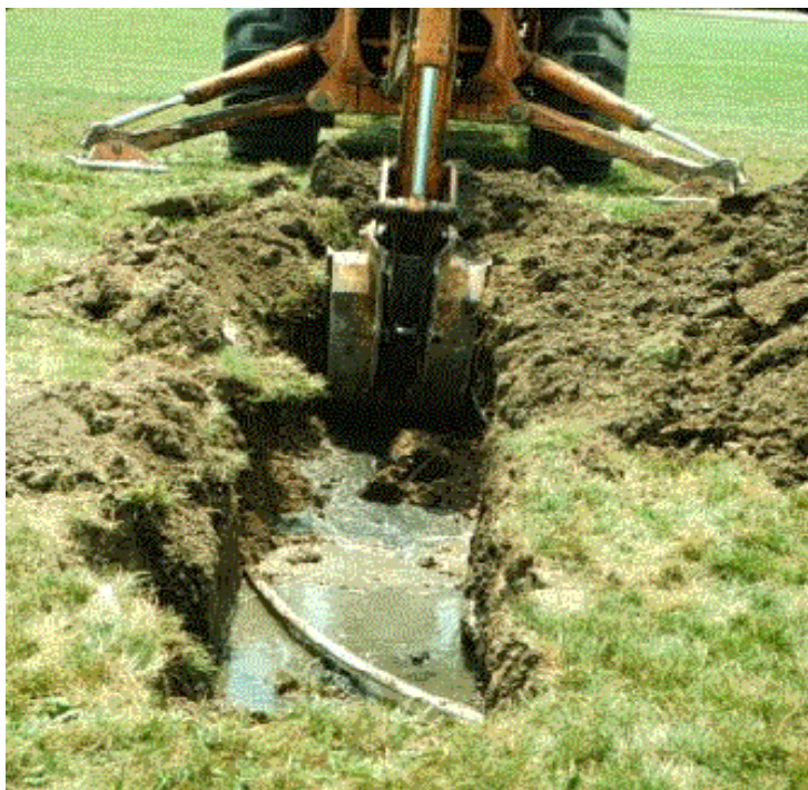
Image 3. Trench Construction
