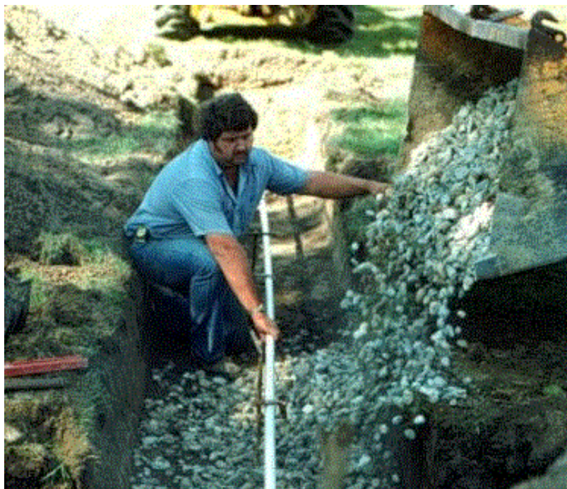
Image 4. Filling Trench with Gravel
