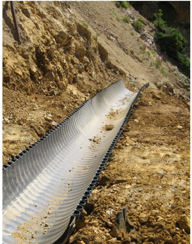
2008 – Installation of permanent portal discharge diversion structure
