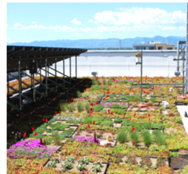
The EPA Region 8 Headquarters' green roof with study plots and instrumentation. The solar panels provide beneficial shade during hot weather. Photo: EPA Region 8.
