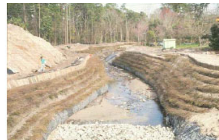
Figure 7.32 VRSS Structure After Construction (Sotir and Fischenich, 2003)
