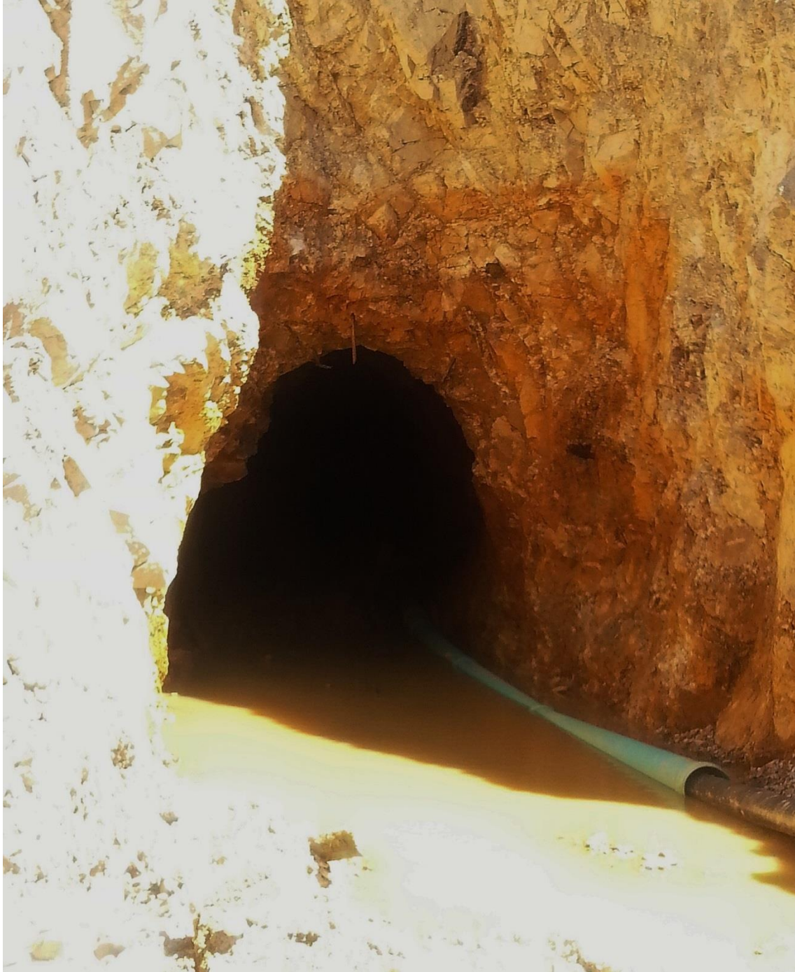
Photo 4 August 18, 2015 – Gold King Mine Level 7 Adit post-blowout
