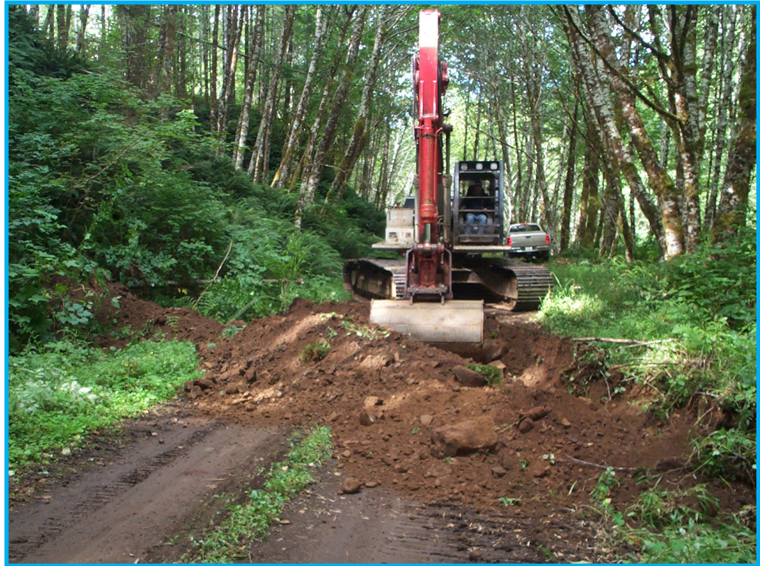
Decommissioning a forest road adjacent to Cruiser Creek; Photo: TEP
