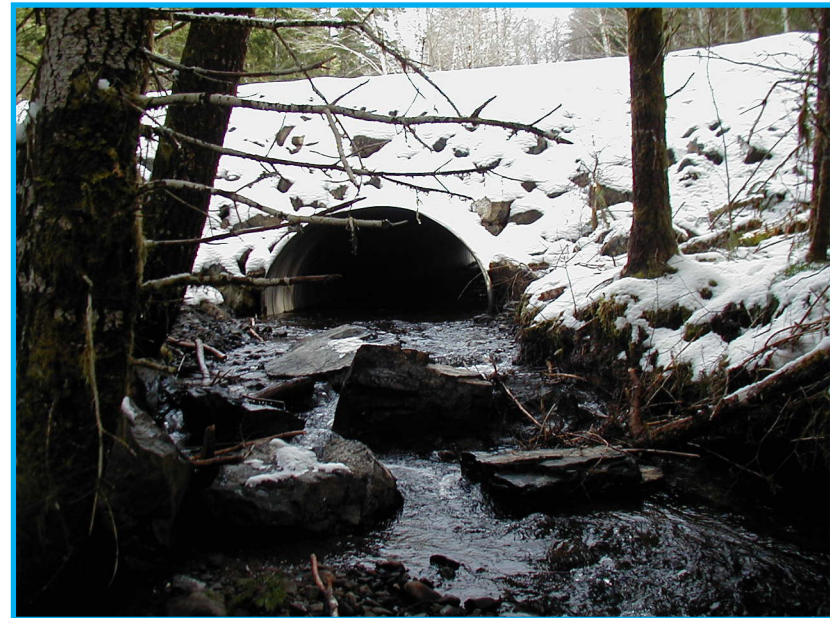
Restored fish passage at one of the Cruiser Creek tributaries; Photo: TEP
