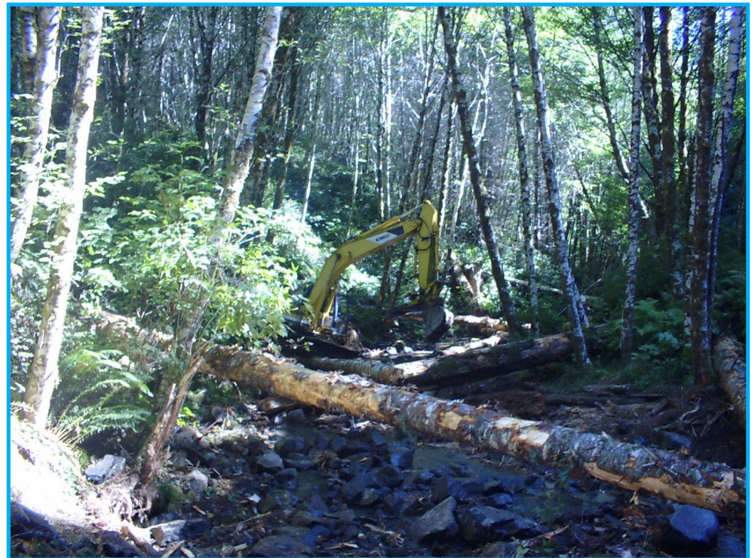
Placing wood and boulder structures in Cruiser Creek; Photo: BLM
