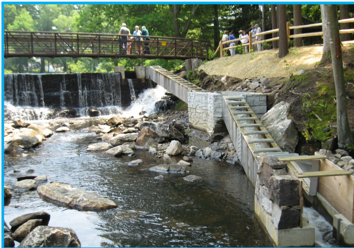
Jordan Millpond Dam and Fishway looking upstream Photo: NOAA
