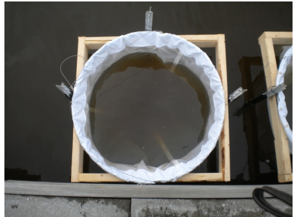
Photograph 40: Pump Effluent in Netting
