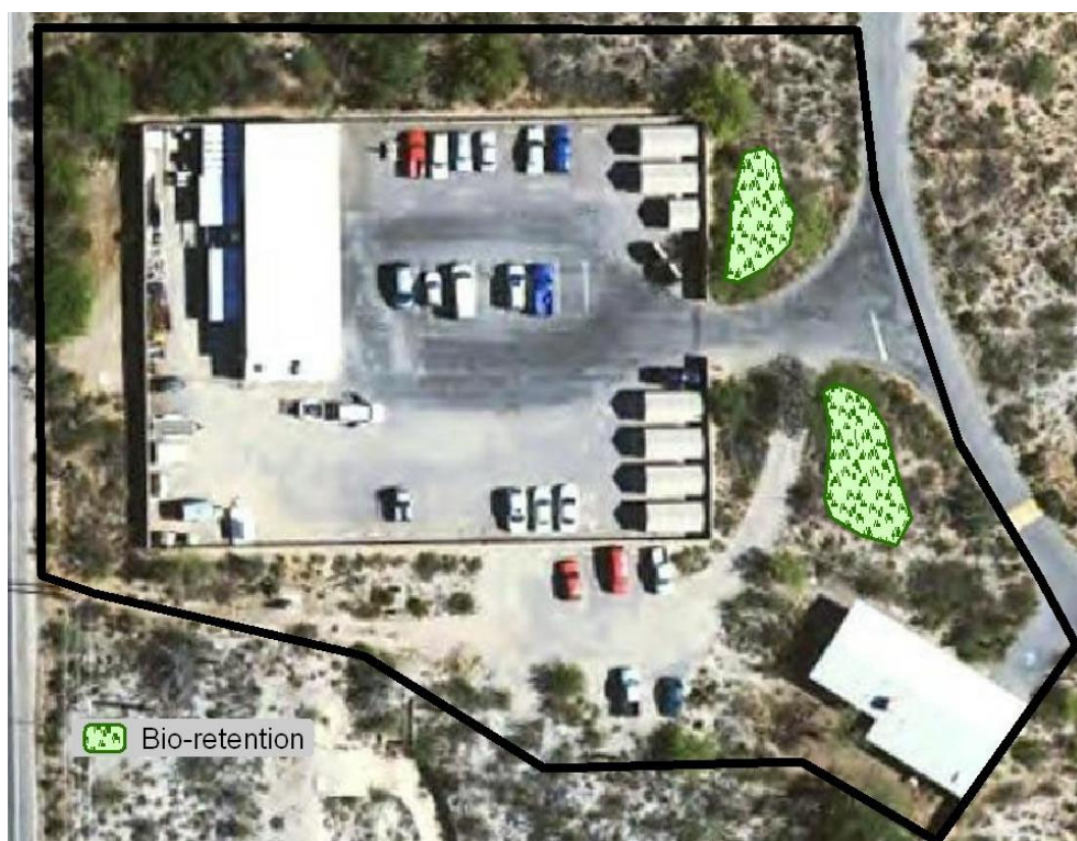
Figure 3A3-7. Actual site and on-site control measures (Phoenix, AZ).
