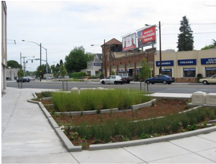
Figure 3A1-6. An urban bioretention system treats sidewalk and road runoff.
