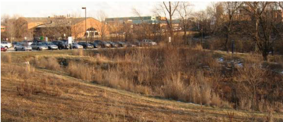
Figure 3A1-21. Stormwater wetland at the University of Maryland, College Park. Runoff from the parking lot enters the wetland from the left, flows in a roughly U-shaped counterclockwise pattern, and discharges via a riser at the top center of the wetland.
