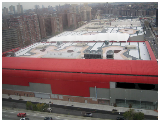
Figure 3A1-4. Rooftop detention being used to control runoff at a commercial property.
