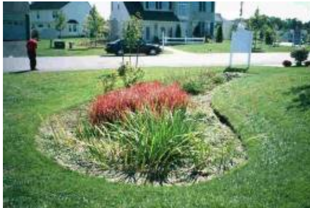
Figure 3A1-5. Bioretention cell for street and yard drainage.
