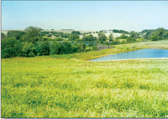
Figure 2. A grade stabilization structure installed in the Lake Binder watershed captures and slows runoff into the lake.
