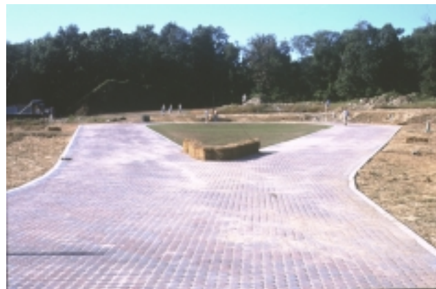
Pervious concrete pavers for roadway in BMP subdivision. Swales will be used instead of curb and gutter (Jordan Cove, Connecticut).
