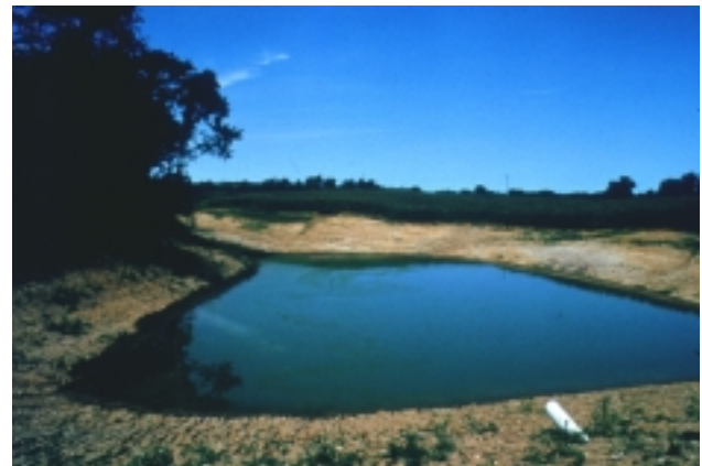
Sediment retention basin (Lake Pittsfield, Illinois).
