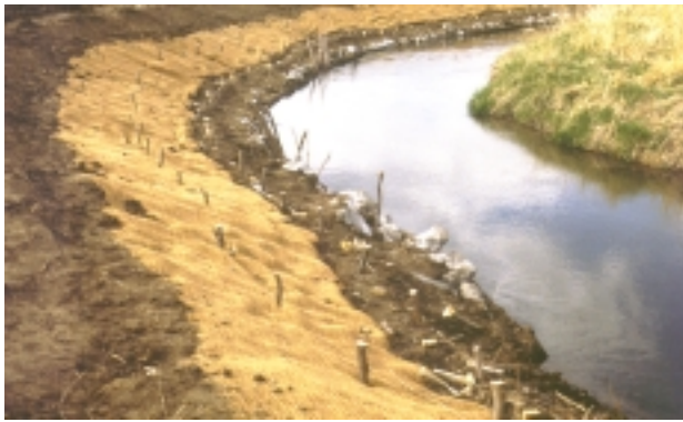
Installation of willow stakes (Elm Creek, Nebraska).
