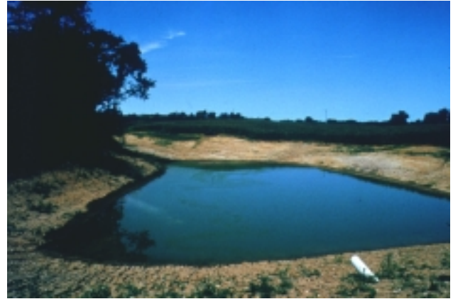
Sediment retention basin (Lake Pittsfield, Illinois).
