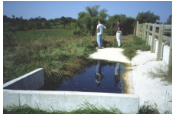
Level spreader for treated barnyard runoff (Otter Creek, Wisconsin).
