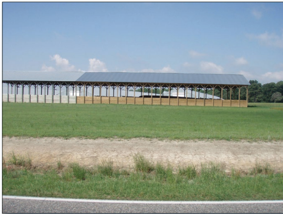
Figure 2. One of the waste storage structures (stacking sheds) installed as part of the CWA section 319 grant. The landowner worked with NRCS to construct a shed using EQIP funds, but needed a larger facility than EQIP allowed. In the end, EQIP funded the initial half of this structure, and CWA section 319 funded the second half at a later date (with the landowner cost-sharing on both).
