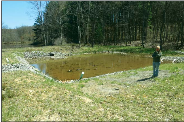
Figure 2. The Bishoff Steel slag bed treatment system, constructed in 2010, adds excess alkalinity to the main stem of Sovern Run.
