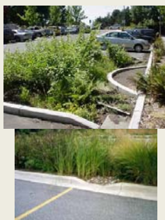
Parking Lot Infiltration Areas
