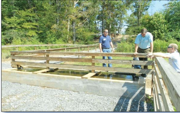
Figure 2. A landowner installed this off-stream watering source to reduce livestock access to surface waters.
