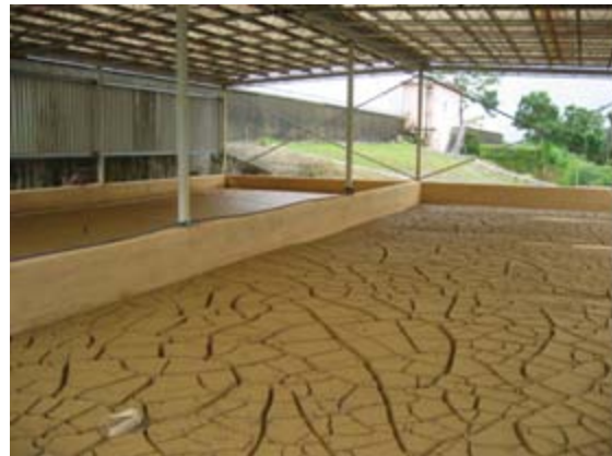
Figure 3-5. Guaynabo WTP Equalization Basin (Left) and Sludge Drying Beds (Right)
