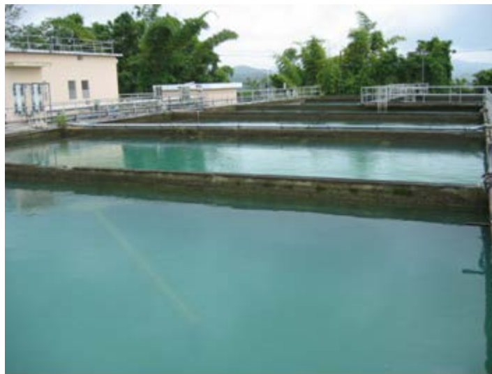
Figure 3-3. Guaynabo WTP Sedimentation Tanks
