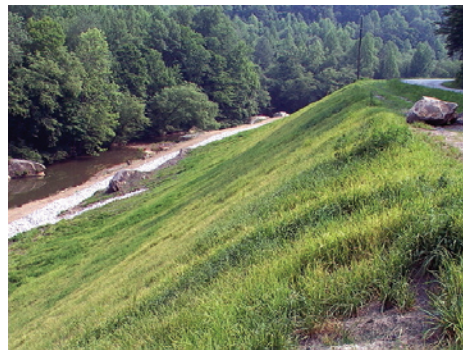
Rock Creek bank after restoration.
