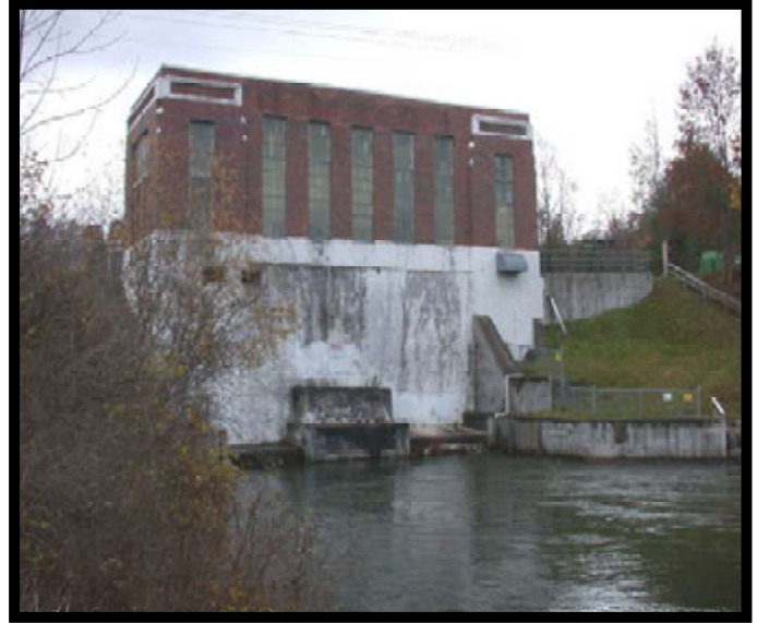
A dam on the Boardman River Source: U.S. Fish and Wildlife Service
