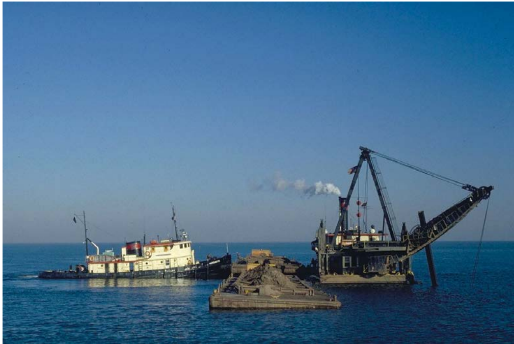
Dredging, Duluth, MN Photograph by: Minnesota Sea Grant
