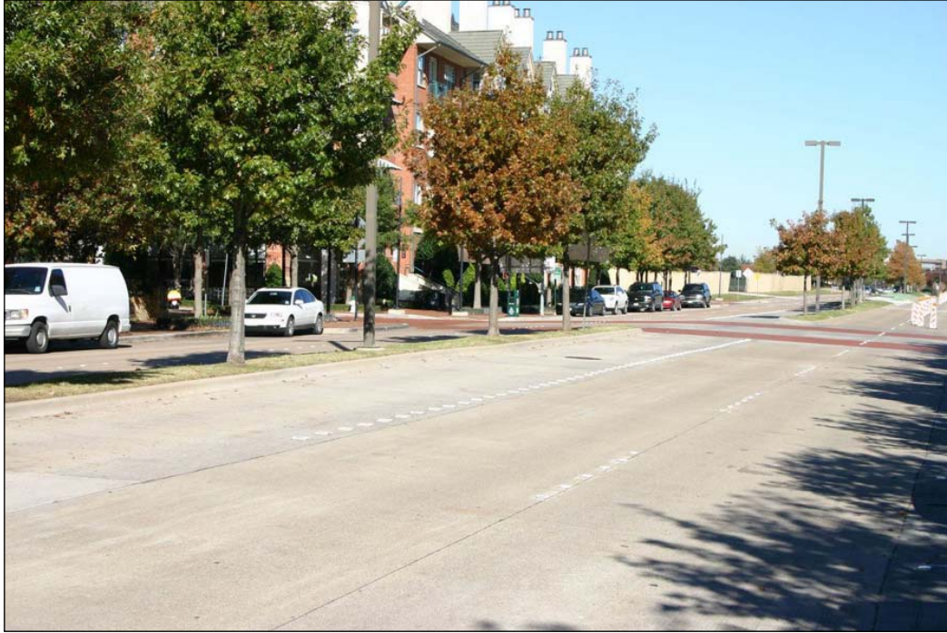
Figure 9.4: An example of 10.5-ft. wide travel lanes on a mixed use arterial in Addison, TX. Source: Kimley-Horn and Associates Inc.
