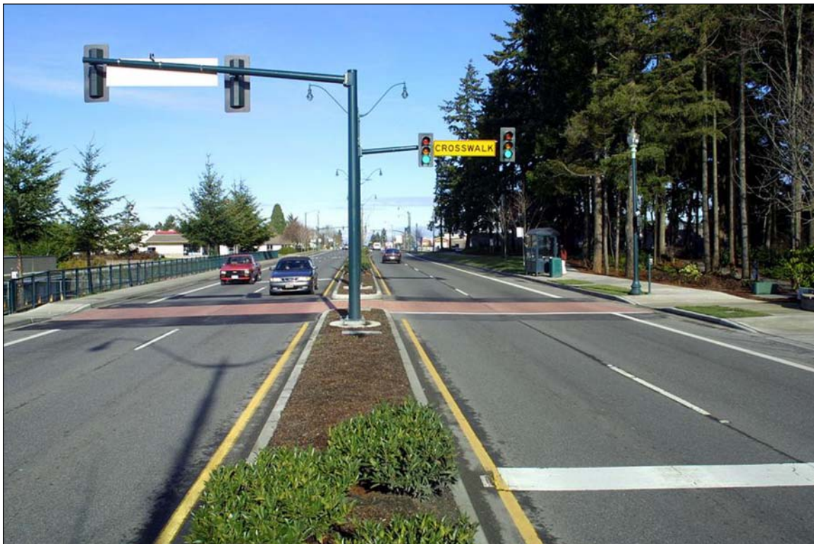
Figure 9.19 Example of a signalized mid-block crossing. Source: Dan Burden, Walkable Communities Inc.
