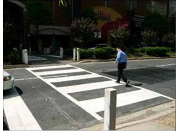
Figure 9.18 Mid-block crossing with pedestrian detection and in-pavement lights. Source: Kimley-Horn and Associates Inc.
