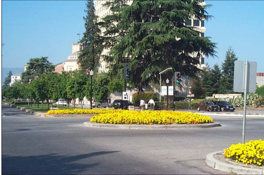
Figure 9.8 A wide median in Mountain View, CA provides attractive landscaping, benches, and other amenities. Source: Kimley-Horn and Associates Inc.
