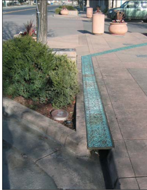
Figure 10.18 Curb extensions may be used as landscaping or hardscape opportunities. This example shows a retrofit curb extension with drainage retained between the extension and the curb. Source: Community, Design + Architecture.
