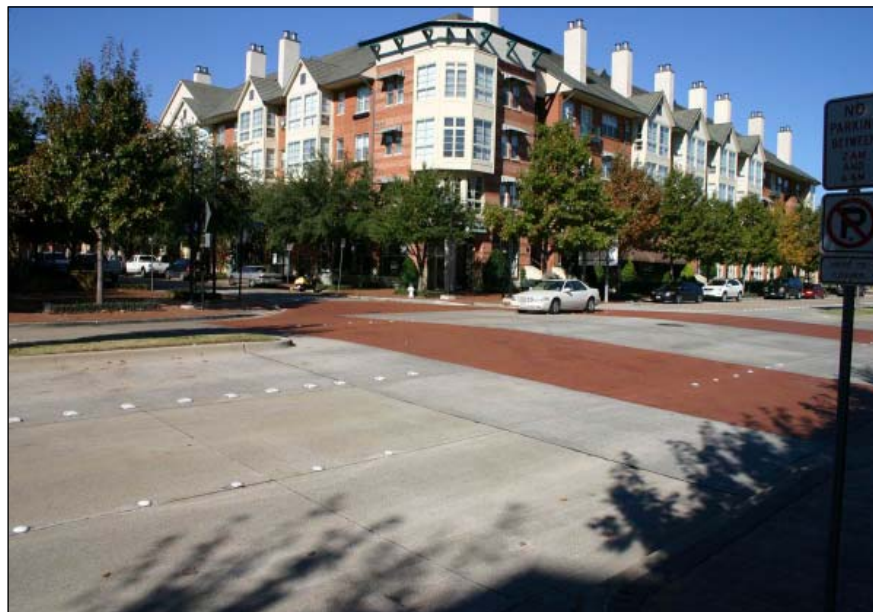
Figure 10.14 Crosswalks with colored bricks contrast with concrete pavement. Painted stripes marking the brick crosswalks increase visibility. Source: Kimley-Horn and Associates Inc.
