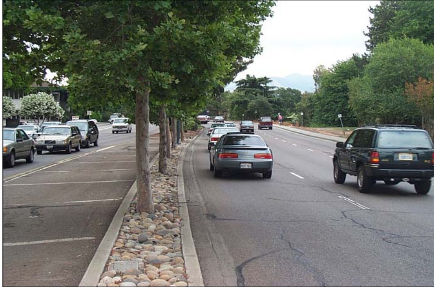
Figure 9.7 Example of trees in median with inadequate horizontal clearance. Median width should be designed to accommodate an 18-in. clearance when trees are mature. Source: Kimley-Horn and Associates Inc.
