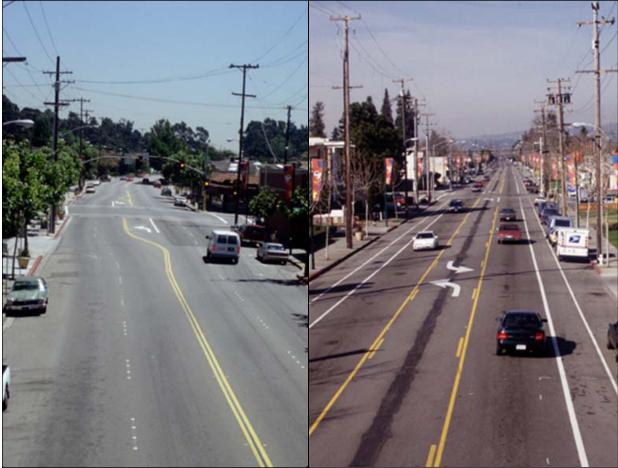
Figure 9.10 A four to three lane conversion to accommodate bicycle lanes, City of San Leandro, CA. Source: City of San Leandro.
