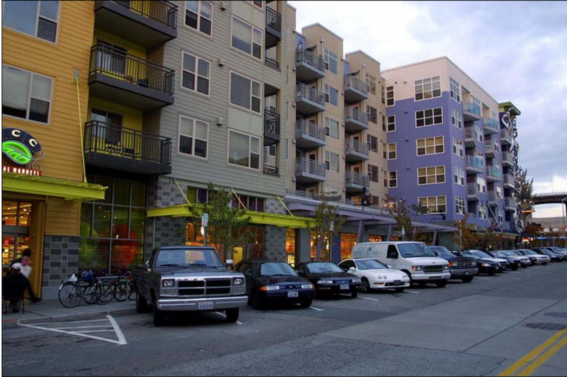
Figure 9.11 Reverse (back-in) angled parking improves driver visibility of bicyclists. Source: Dan Burden, Walkable Communities Inc.
