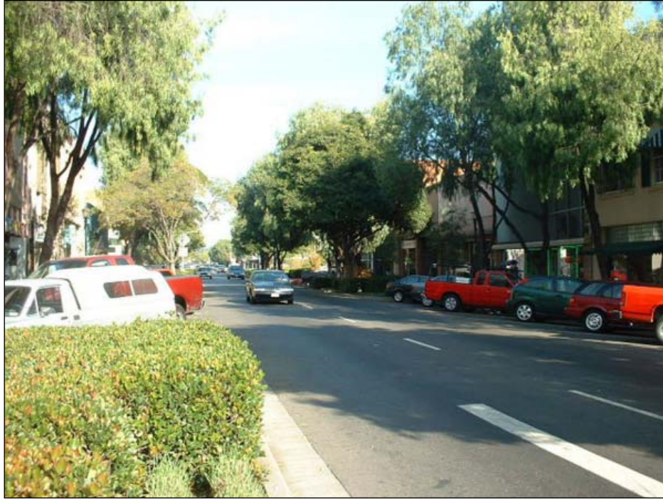
Figure 9.12 Angled parking on a retail-oriented main street in Hayward, CA. Source: Kimley-Horn and Associates Inc.
