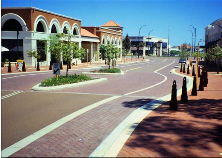
Figure 10.16 A mid-block crossing with a flush curb in Australia. Pedestrians are separated from passing vehicles with bollards. Source: Community, Design + Architecture.
