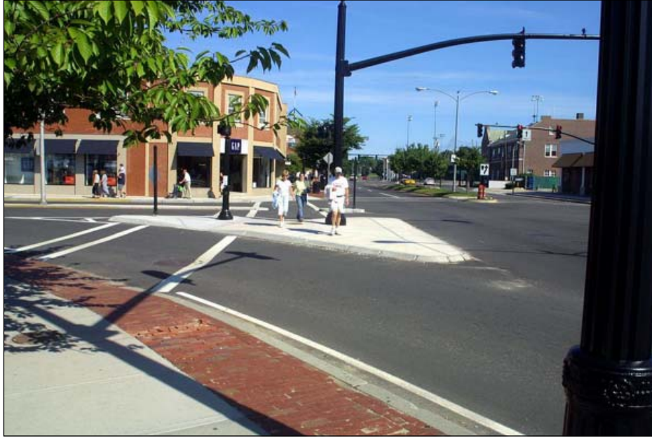
Figure 10.9 A channelized right turn lane typically provides a pedestrian refuge island and an uncontrolled crosswalk. Source: Dan Burden, Walkable Communities Inc.
