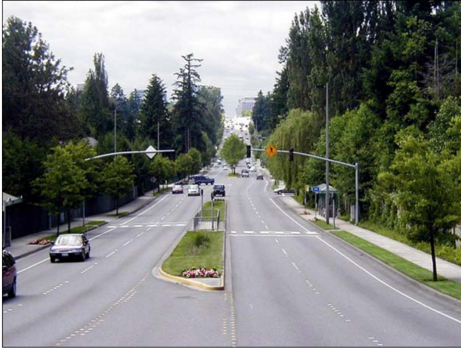
Figure 9.15 Midblock crosswalks provide opportunities to cross streets with long distances between intersection crossings. Source: Dan Burden, Walkable Communities Inc.
