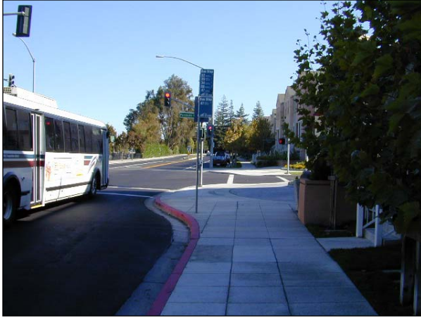
Figure 9.22 A typical bus turnout on an arterial avenue. Source: Kimley-Horn and Associates Inc.
