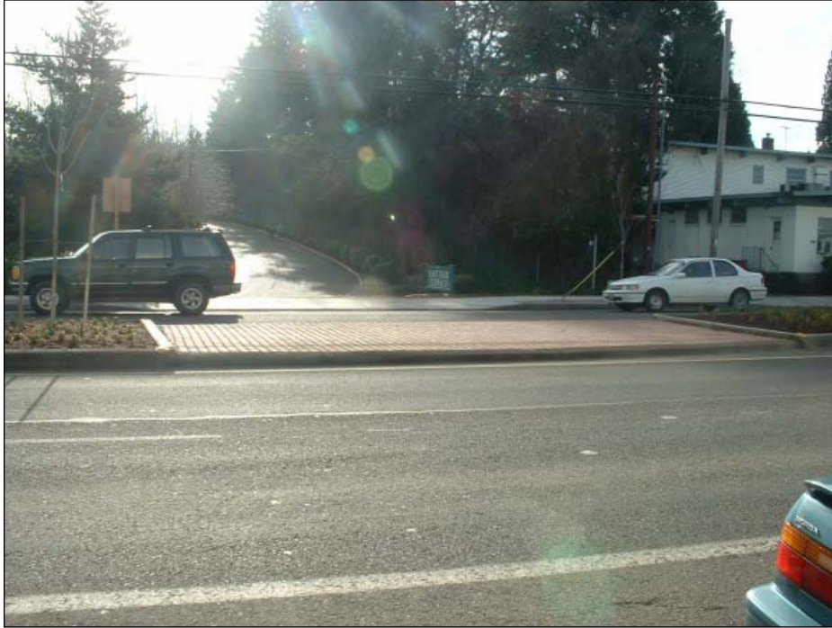
Figure 9.2 A mountable median allows emergency vehicles to access streets otherwise difficult to access because of access management. Source: Kimley-Horn and Associates Inc.
