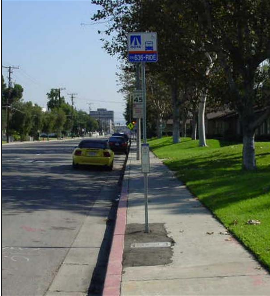
Figure 9.21 Parking restrictions at a bus stop using a red curb. Source: Kimley-Horn and Associates Inc.
