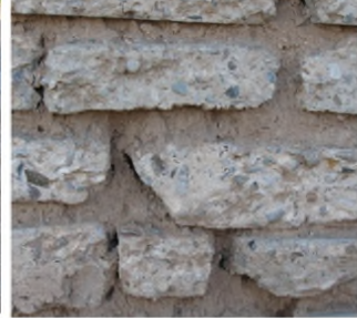
RECYCLED CONCRETE WALL
