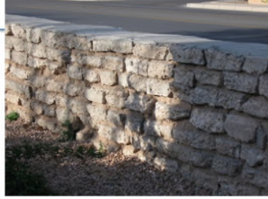
RECYCLED CONCRETE WALL
