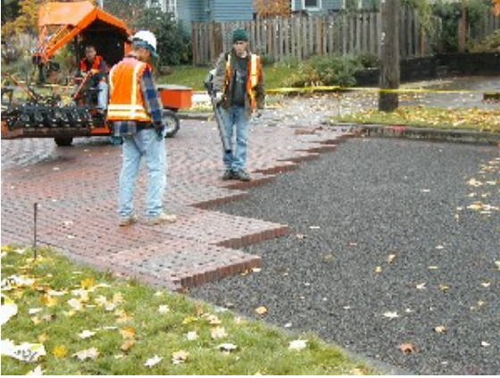
Figure 1: Project during construction
